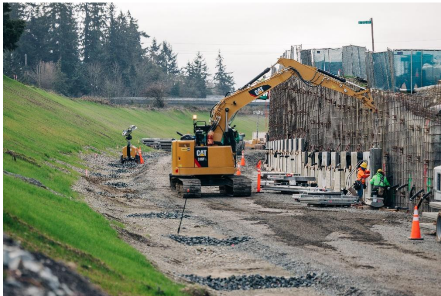
Figure B5-6 Retained-Cut Construction (Typical)
