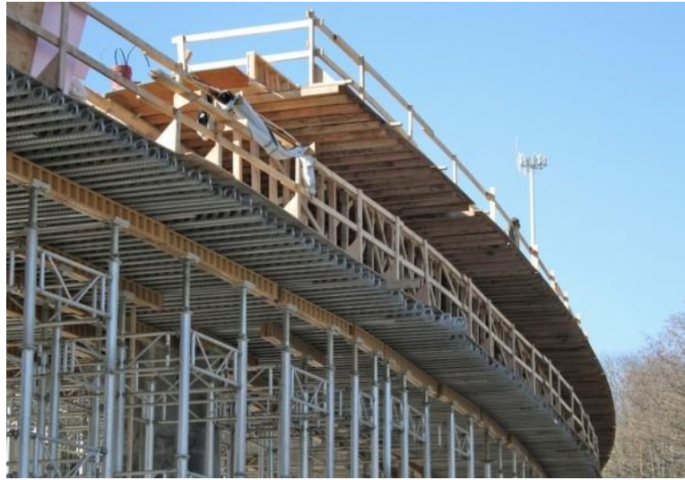
Figure B5-2 Elevated Guideway Construction Showing Falsework (Typical)
