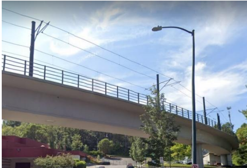
Figure B3-7 Typical Overhead Catenary System
