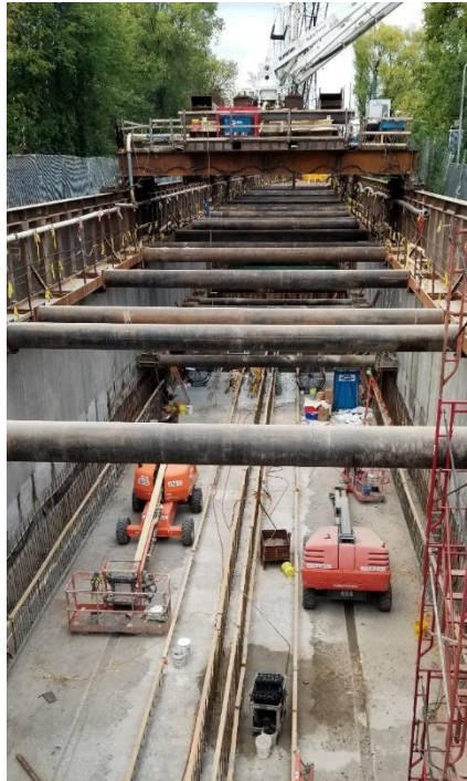
Figure B5-7 Cut-and-Cover Construction (Typical)
