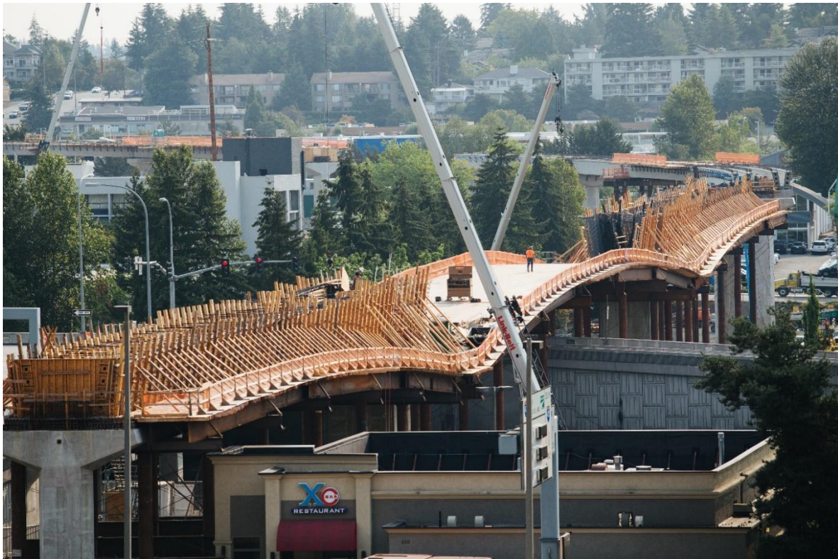
Figure B5-5 Elevated Guideway Construction Over Roadways (Typical)
