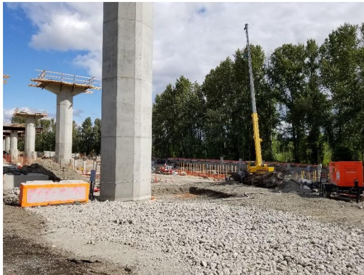
Figure B5-1 Construction of Guideway Columns (Typical)
