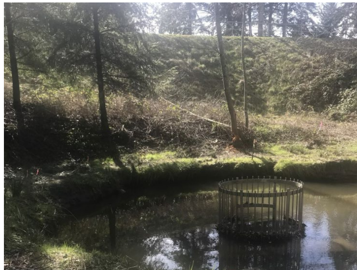
Figure 4.8-2 Siphoned Culvert at Southwest Genesee Street Dam Outlet
