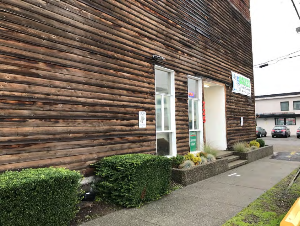
Photo 1. Subject property southeast corner of the building.
