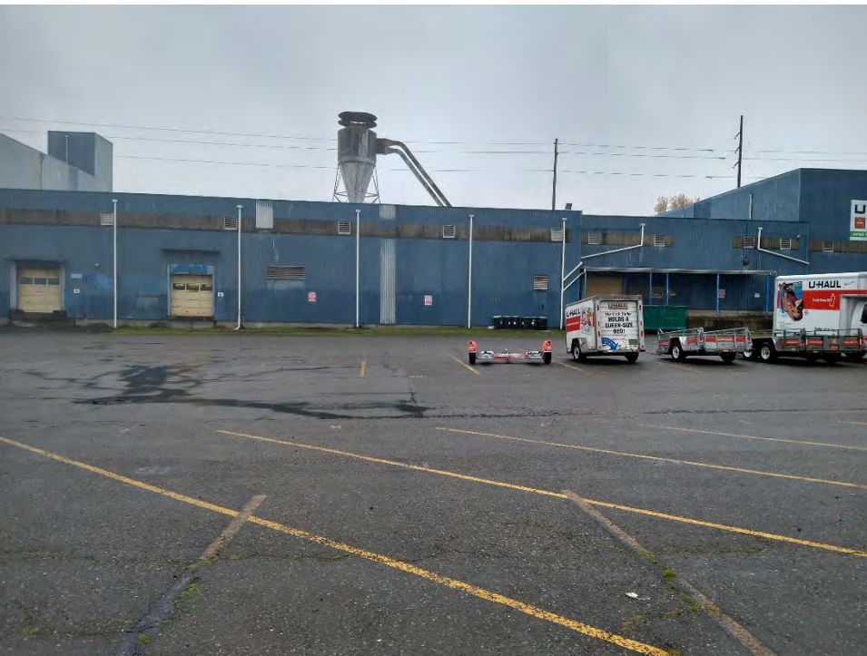
Photo 2. Subject property and adjacent property north. Non-hazardous waste drums located north of the building.
