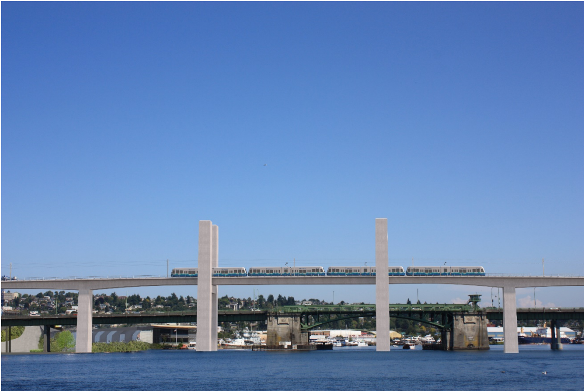
Figure 3-8c. KOP B-8: Elevated 15th Avenue Alternative (IBB-3)
