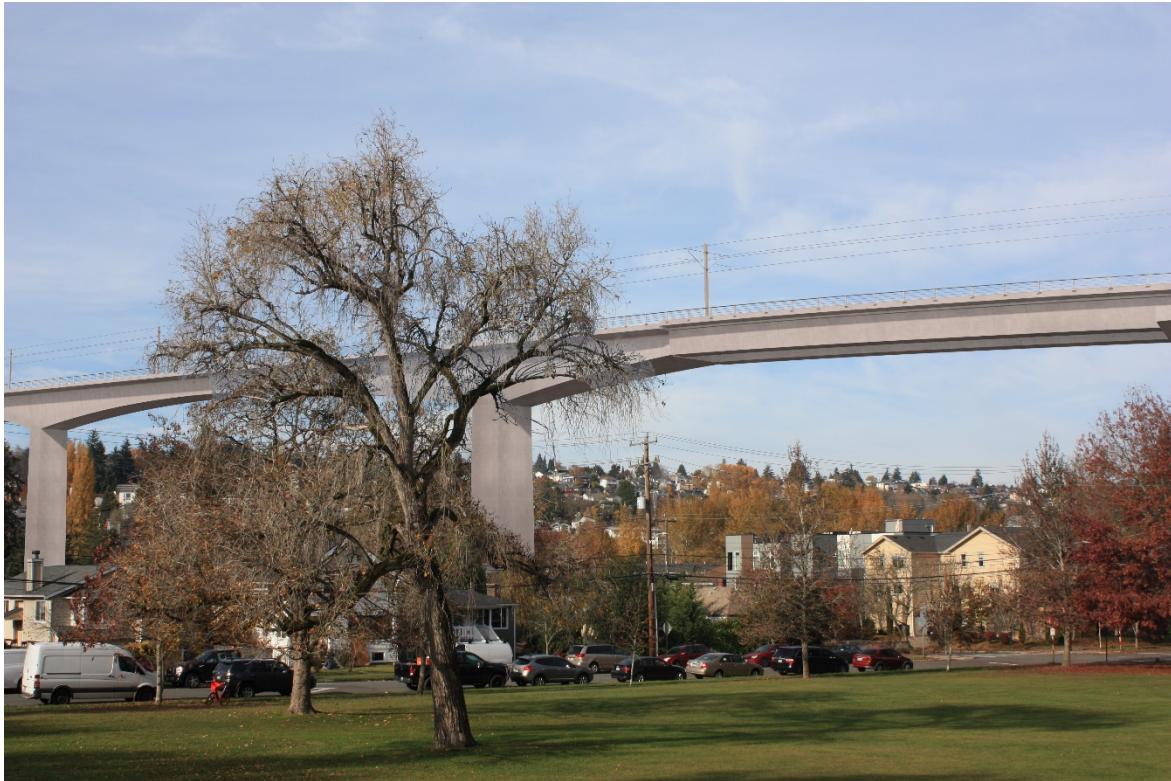
Figure 2-6d. KOP WS-6: Delridge Way Station Alternative (DEL-3)
