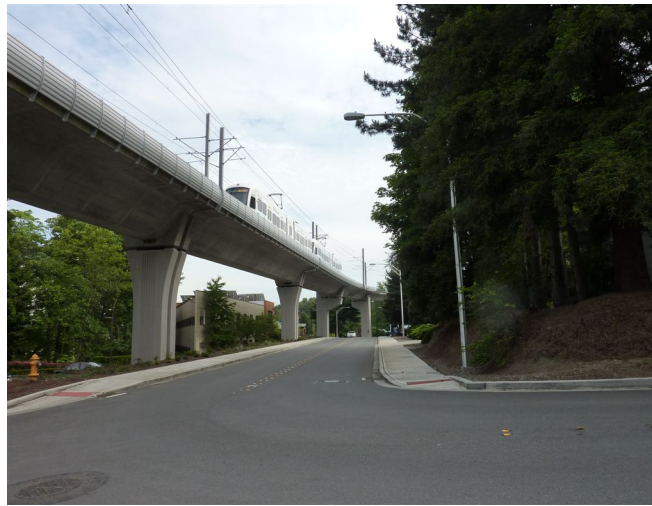
Figure 4-2. Sound Wall on Elevated Guideway
