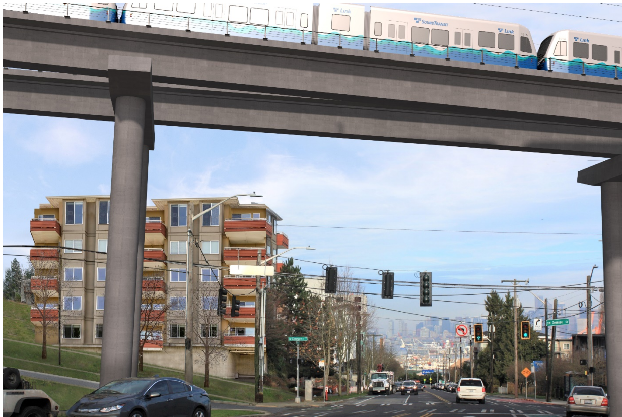
Figure 2-10d. KOP WS-10: Delridge Way Station Alternative (DEL-3)
