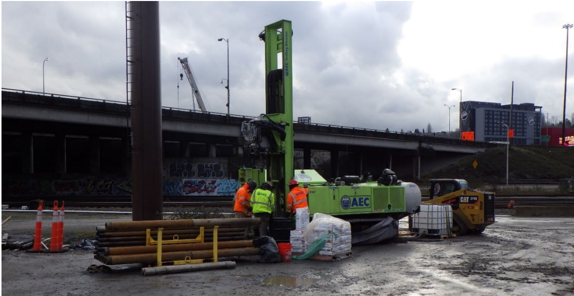
Figure 5-2 Archaeological Boring Using a Sonicore at AB-8
