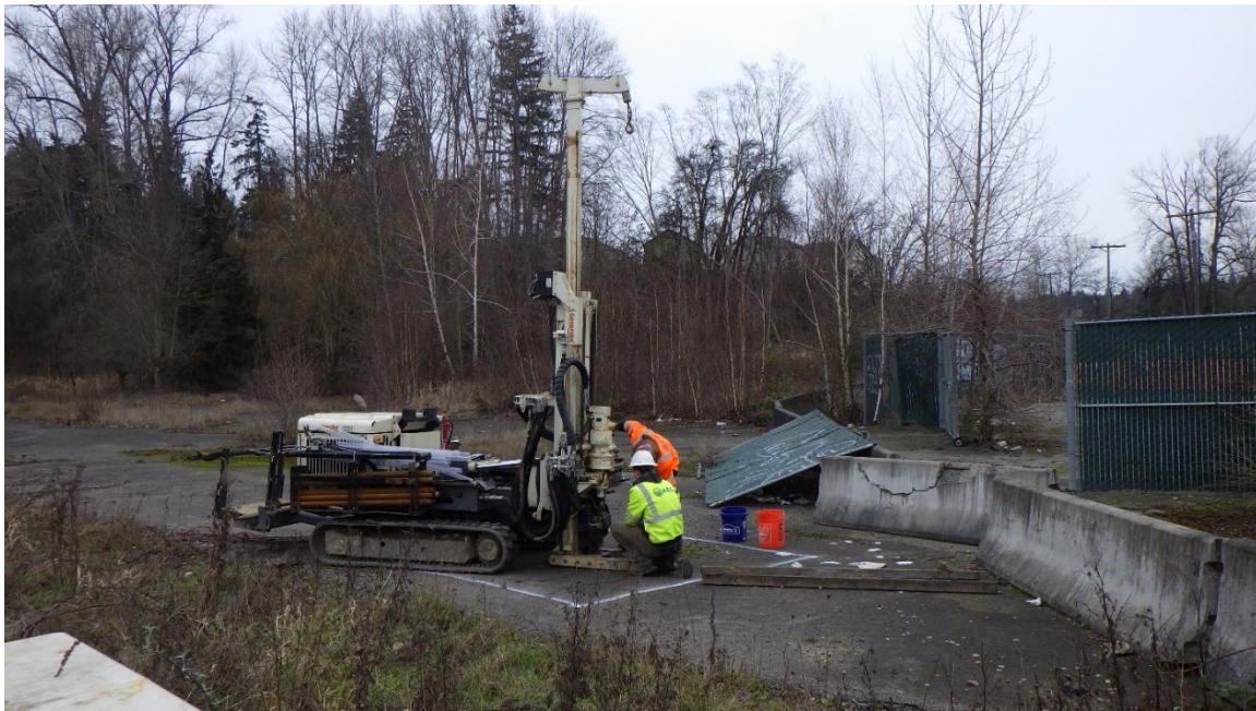
Figure 5-1 Archaeological Boring Using a Geoprobe at AB-20
