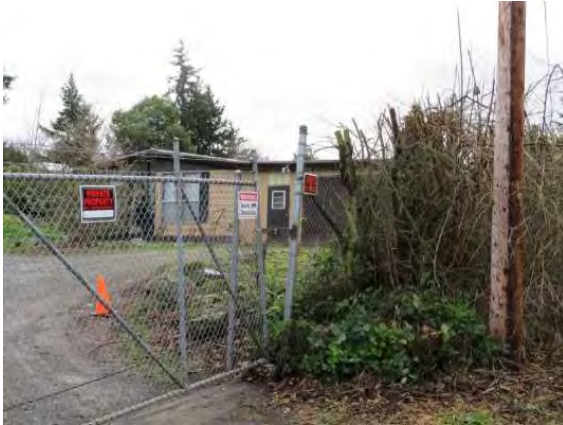
36200 16th Avenue S, view southeast.jpg
