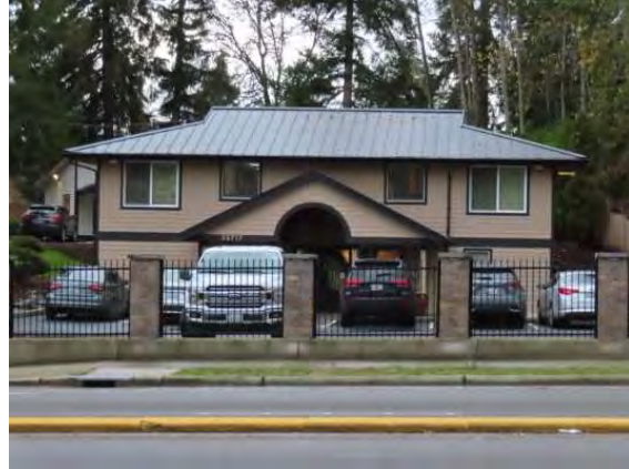
35717 Pacific Highway S, view east.
