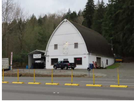
37205 Pacific Highway S, view southwest.
