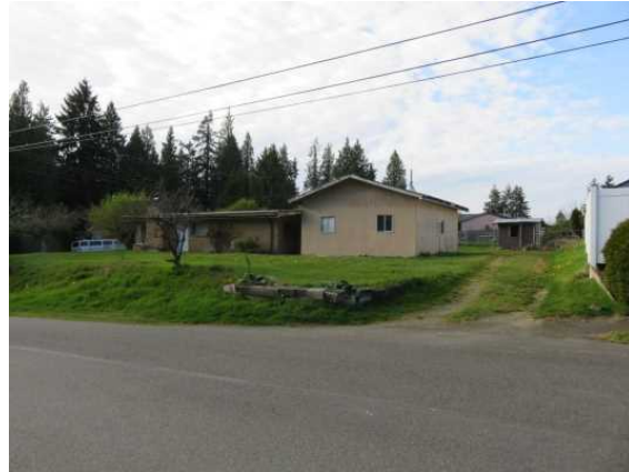
2206 S 330th St, view northwest
