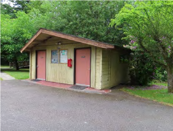
36605 Pacific Highway, natatorium, view east.
