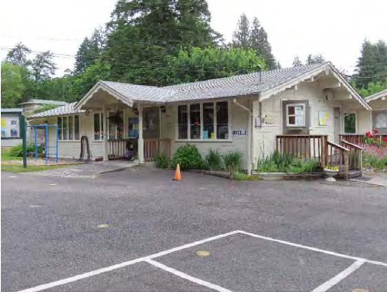
36605 Pacific Highway, Classrooms 4, view south.
