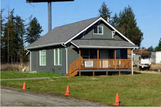
320 Birch Street, view north
