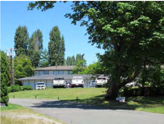
1220 S 356th Street, northern building (background), view northeast
