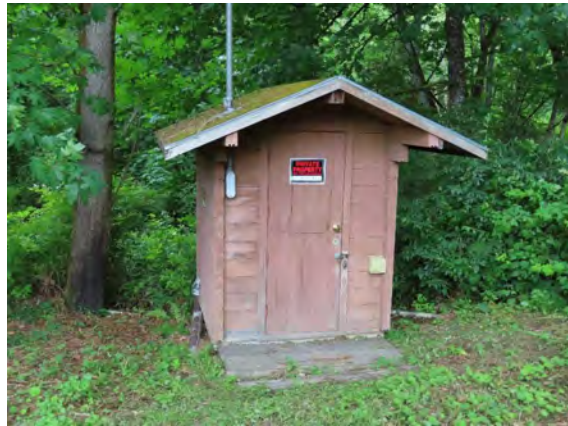
36605 Pacific Highway, Classrooms 6 and 7, wellhouse, view west.
