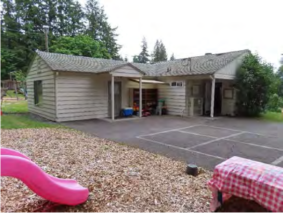
36605 Pacific Highway, Classrooms 6 and 7, view southeast.
