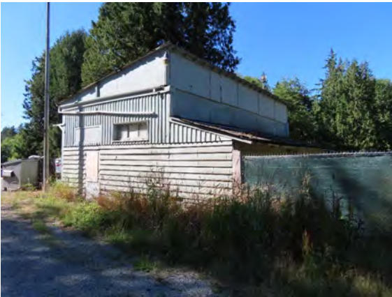
726 S 356th Street, outbuilding, view northwest.
