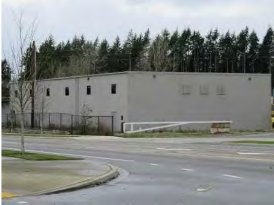
1393 S 351st Street, view northwest.jpg
