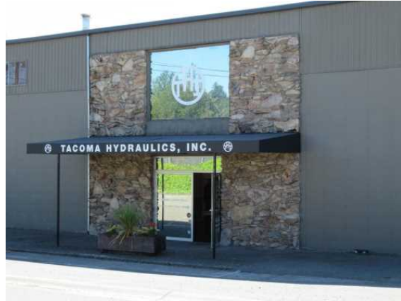
405B Porter Way main entrance, view southwest
