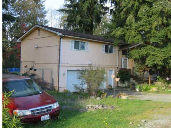
2238 S 333rd St, view northeast
