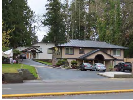
35800 Pacific Highway S, view east.
