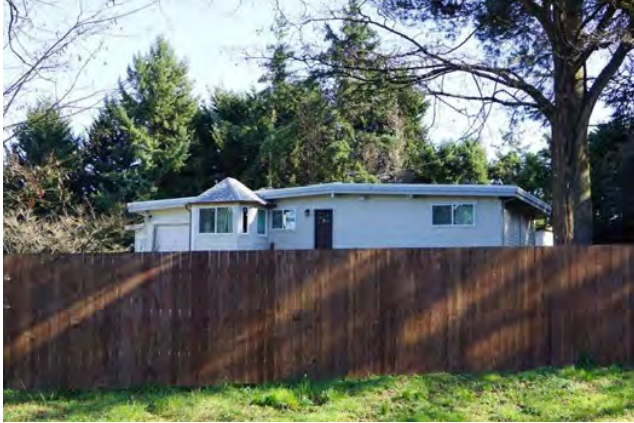
37540 8th Avenue S, view northeast
