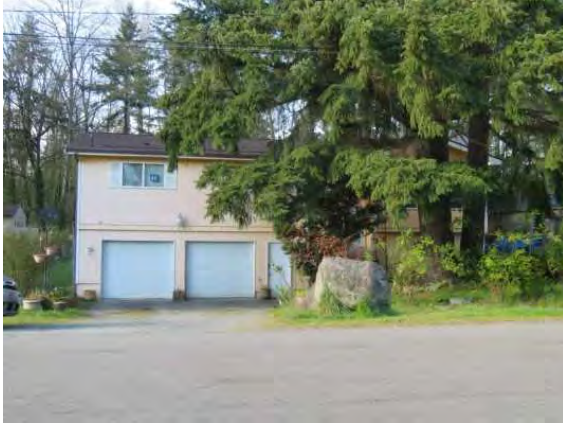
2238 S 333rd St, view north
