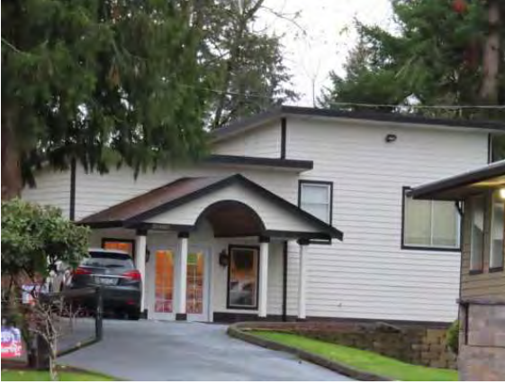
35800 Pacific Highway S, view east.
