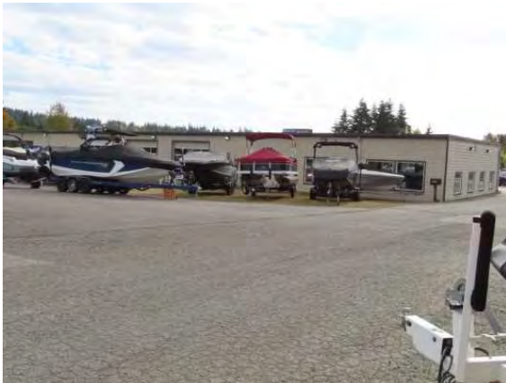
7700 Pacific Highway E, view southeast.
