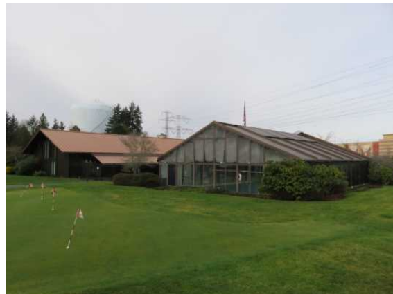
Clubhouse and attached pool house located at 2101 S 324th Street, view northwest.JPG
