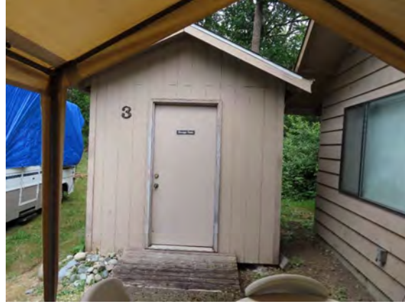
36605 Pacific Highway, conference room storage, view northeast.
