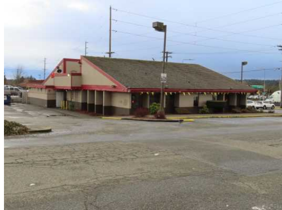
34726 16th Avenue S, view southwest.
