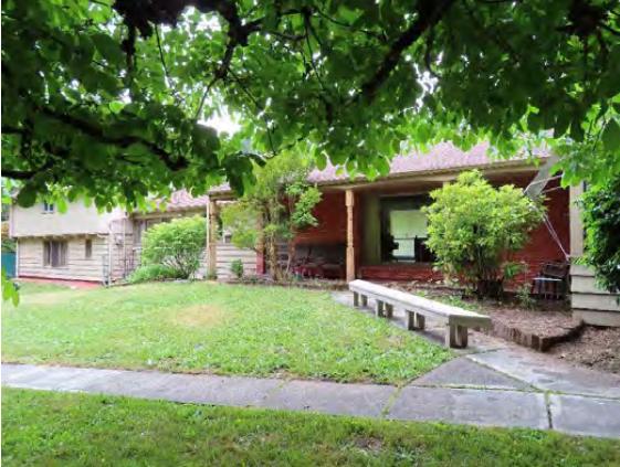
36605 Pacific Highway, residence, view west.
