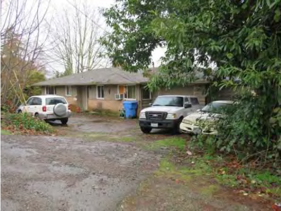
1123 70th Ave. E, view northeast
