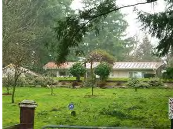
36920 12th Avenue S, King County Assessor, undated
