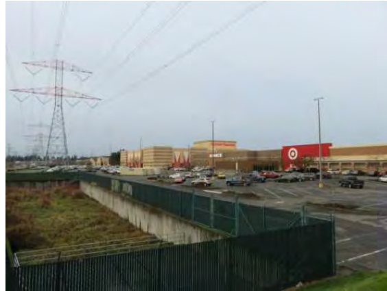
1706 S Commons, view with retention pond, view northwest.JPG
