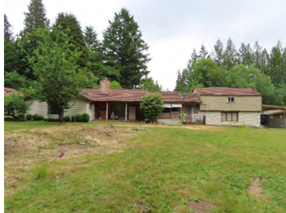
36605 Pacific Highway, residence, view southeast.
