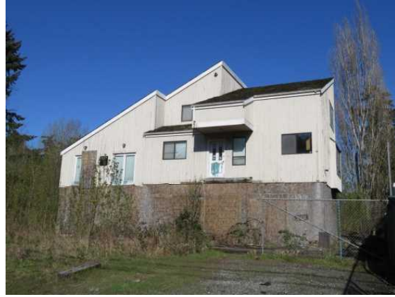
7808 Pacific Hwy, view northeast
