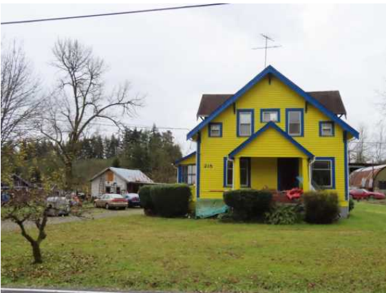
215 S 373rd Street, view south.
