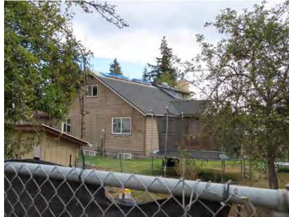
8324 Pacific Highway E, view southeast.
