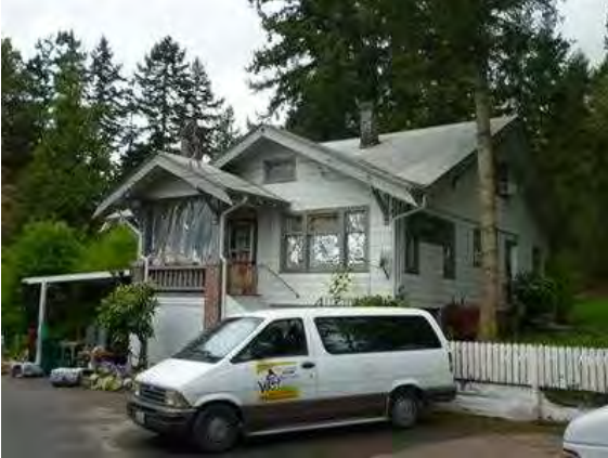
36903 Pacific Highway S, undated, courtesy of the King County Assessor.
