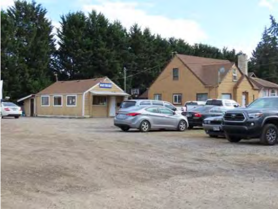
8410 Pacific Highway E, view southeast.
