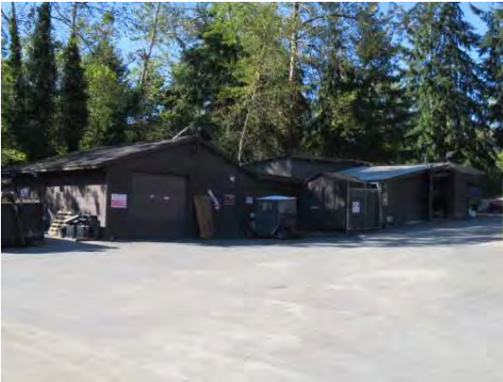
Belmor Mobile Home Park, garage and maintenance
