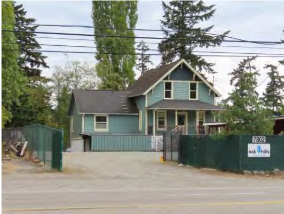
7802 Pacific Highway E, view southeast.
