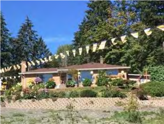
36815 Pacific Highway S, undated, courtesy of the King County Assessor.
