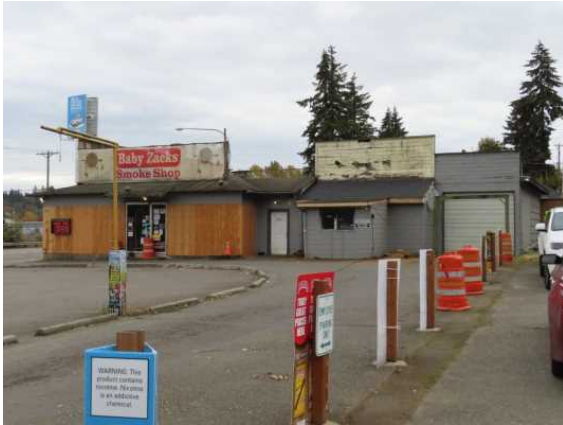
7403 Pacific Highway E, view southeast.
