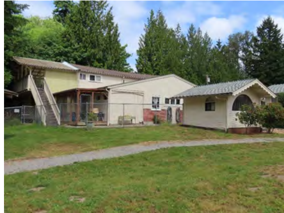
36605 Pacific Highway, Classrooms 1, 2, and 3, view north.
