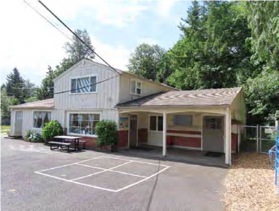
36605 Pacific Highway, Classrooms 1, 2, and 3, view south.
