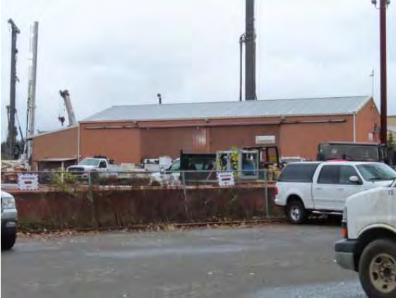
1200 S 356th Street, view northeast.
