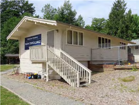
36605 Pacific Highway, Classrooms 5, view southwest.
