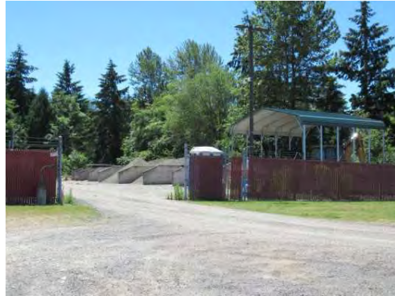
Water Tower structures along S 324th Pl, view southwest
