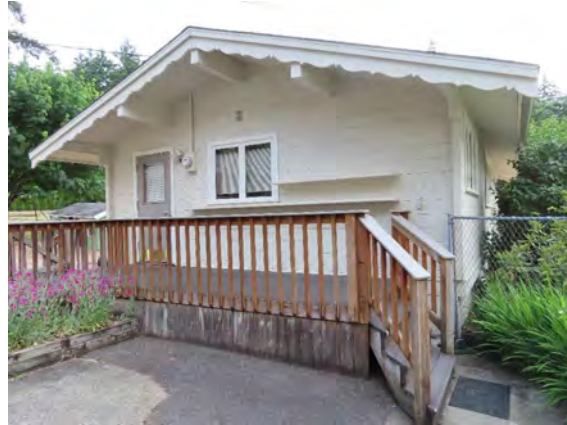
36605 Pacific Highway, Classrooms 5, view east.
