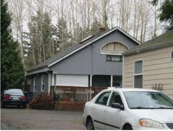
2230 S 336th Street, view northeast.JPG
