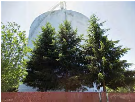
Water Tower along S 324th Pl, view southwest
