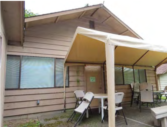
36605 Pacific Highway, conference room, view southeast.
