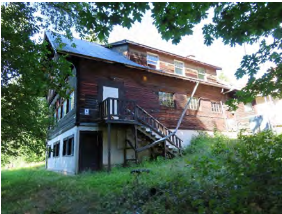
726 S 356th Street, view northeast.
