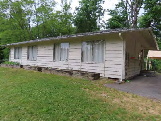
36605 Pacific Highway, Classrooms 8 and 9, view north.
