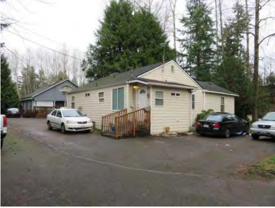
2234 S 336th Street, view northeast.JPG
