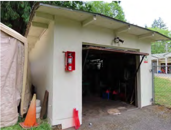
36605 Pacific Highway, Classrooms 6 and 7, garage, view north.
