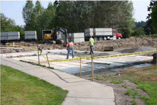
installing empty liners
