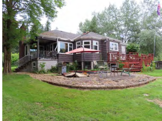
36928 Pacific Highway S, view northwest.
