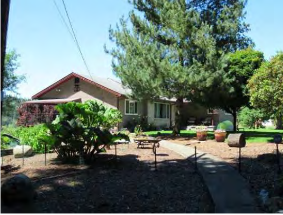
700 S 376th St, view northwest
