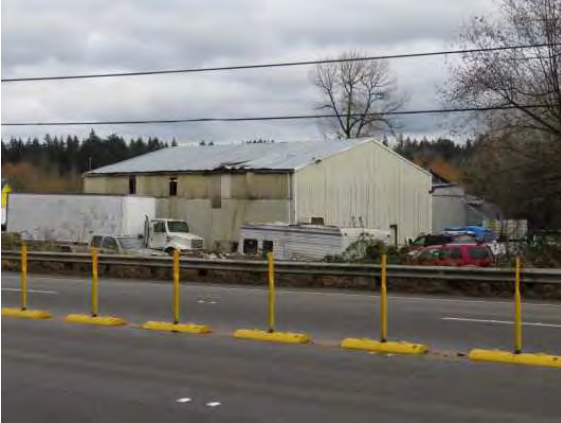
215 S 373rd outbuilding, view northeast.
