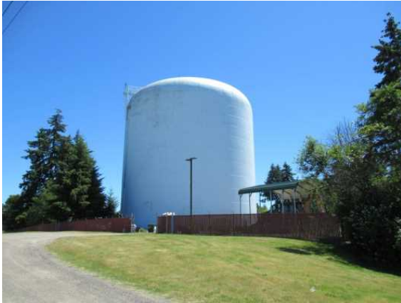
Water Tower along S 324th Pl, view southeast
