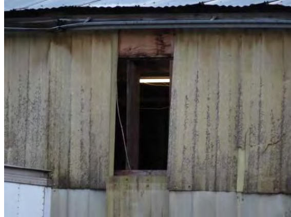
215 S 373rd outbuilding (uncovered opening east elevation)
