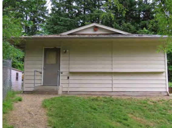
36605 Pacific Highway, Classrooms 8 and 9, view east.
