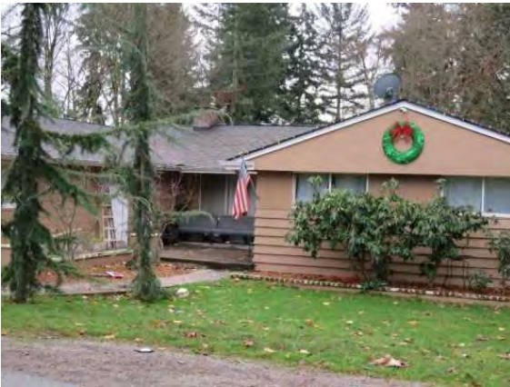
1649 S 359th Street, façade, view south.
