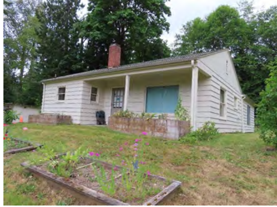
36605 Pacific Highway, Classrooms 6 and 7, view north.
