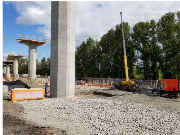
Figure 2-65. Construction of Guideway Columns
