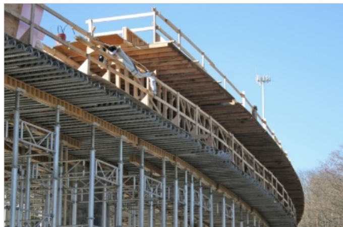
Figure 2-66. Construction of Elevated Guideway Showing False-work
