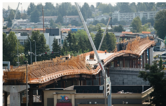
Figure 2-67. Construction of Elevated Guideway Over Roadways
