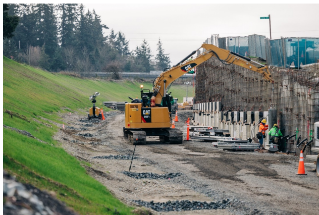
Figure 2-68. Retained-cut Construction
