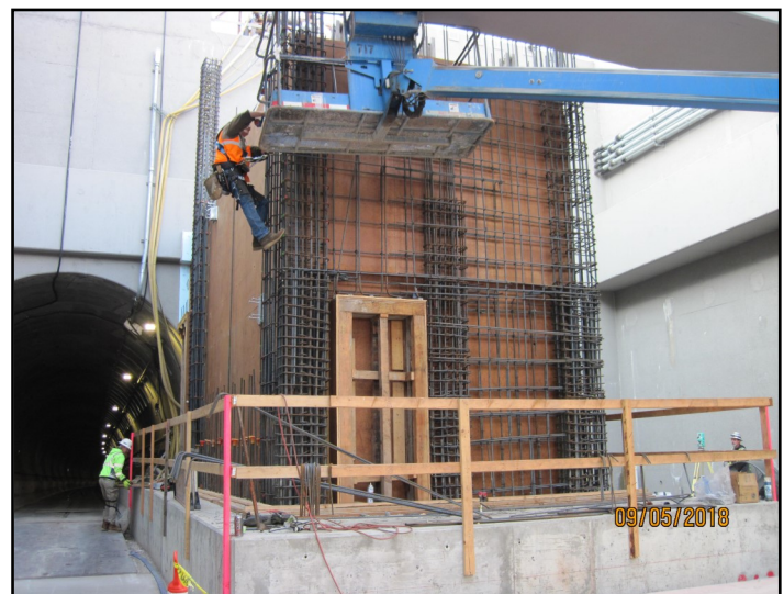
North rebar mat completion.
