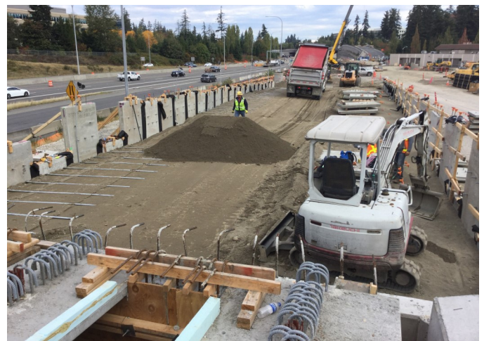
Work Area 3: MSE Wall Backfill along SR520.
