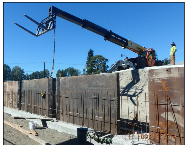
Setting 130th Station south retaining wall panel
