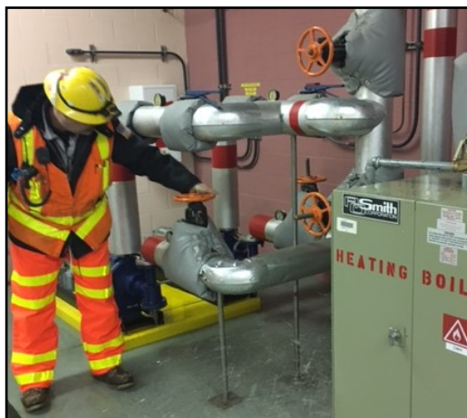
Opening foam valve during commissioning test in tunnel foam room.
