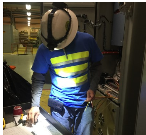
Electrical punch list work: labeling control panel wires.
