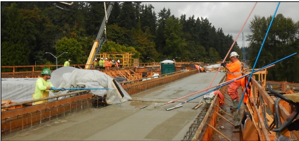
E320 South Bellevue - Placing concrete into track slabs
