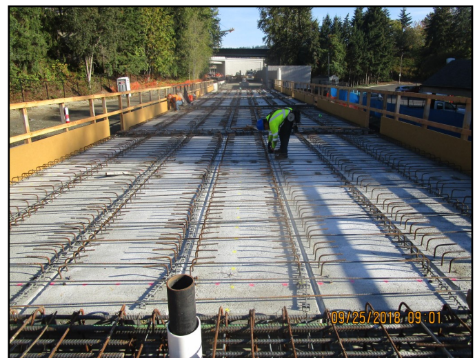
Track rebar installation. (Area 4)
