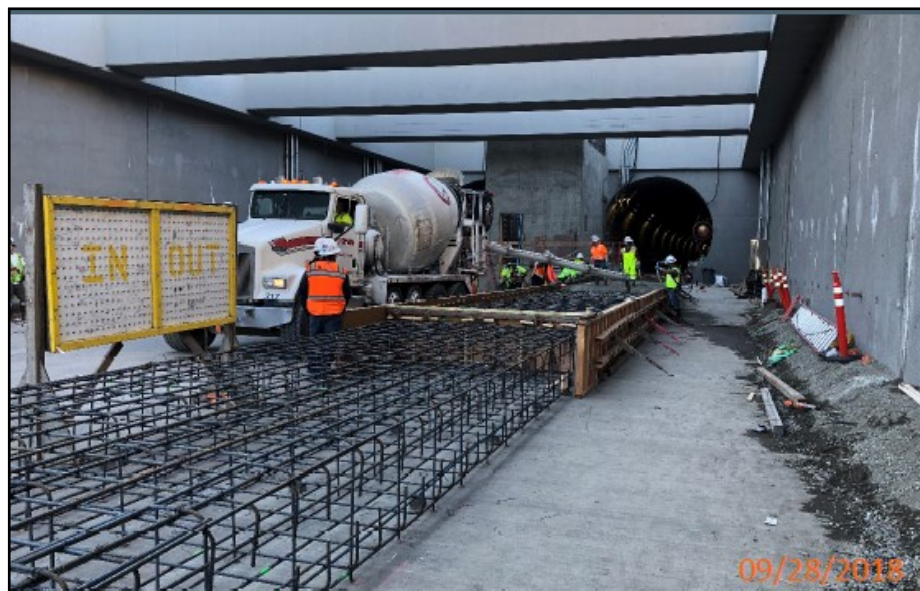
N180 — Placing Southbound Track Slab at Maple Leaf Portal.
