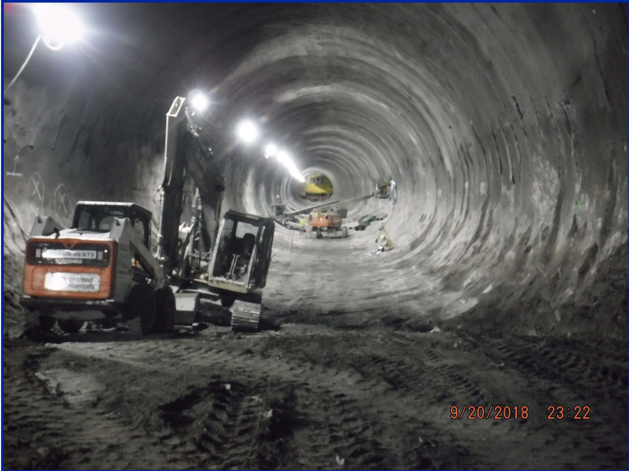
Applying smoothing layer to the tunnel invert at the Downtown Bellevue Tunnel.
