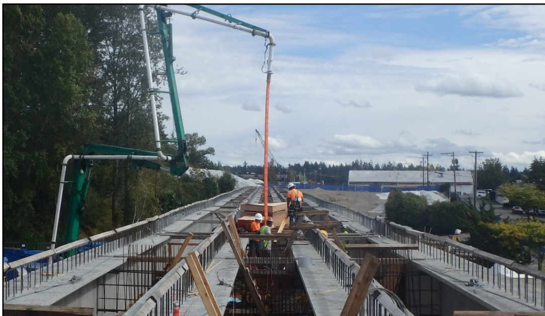
E340 Bel-Red: Placing concrete for girder stops.
