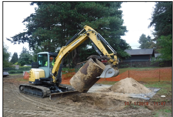
L115 demolition U/G storage tank removal
