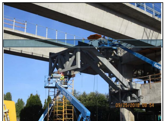
Welding Emergency Stair over Roadway.
