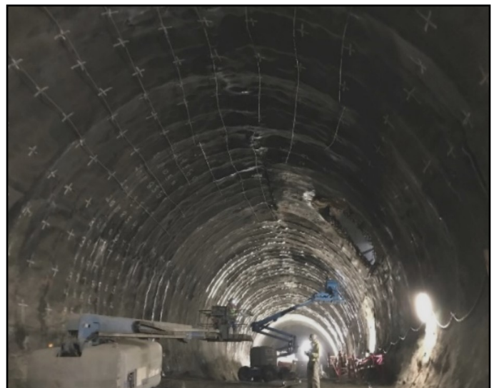
Dowell installation in Tunnel crown in expanded tunnel section
