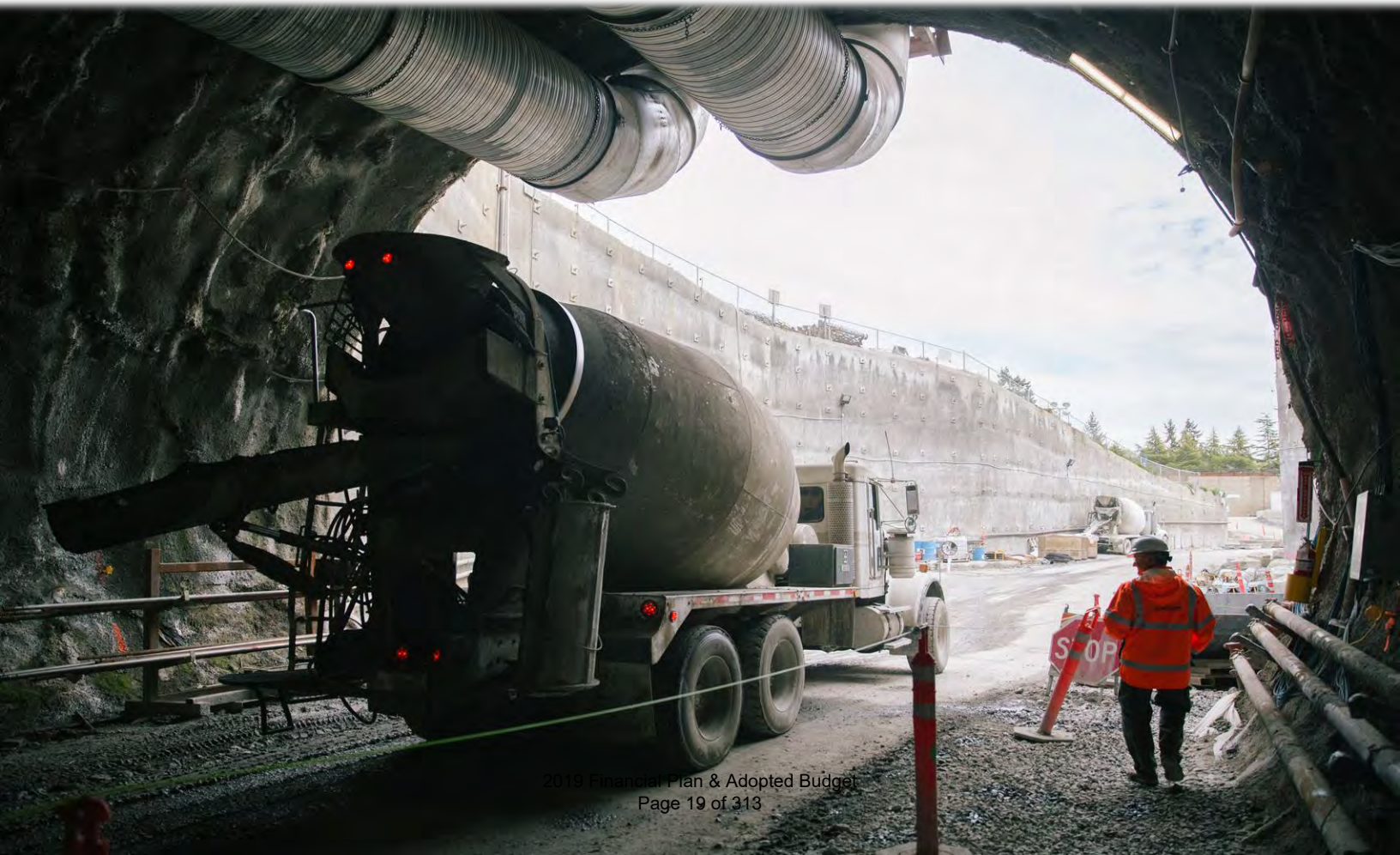
Downtown Bellevue Tunnel
