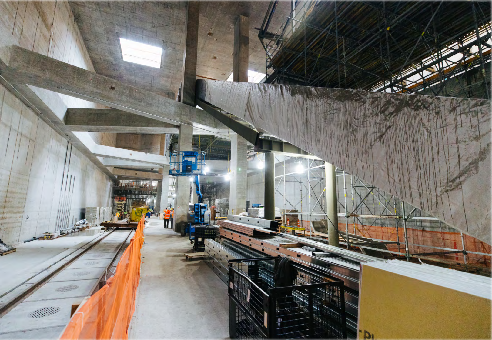
University Station District under construction
