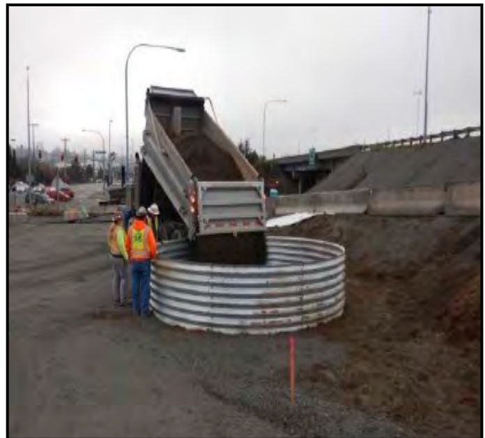
Crew Filling Drill Pad A10 Multi Plate Caisson S
