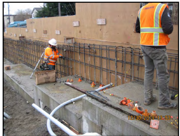
Placing rebar for MLP Southeast screen wall.
