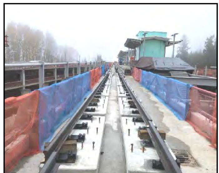
Plinth and track work on elevated guideway at station and garage.
