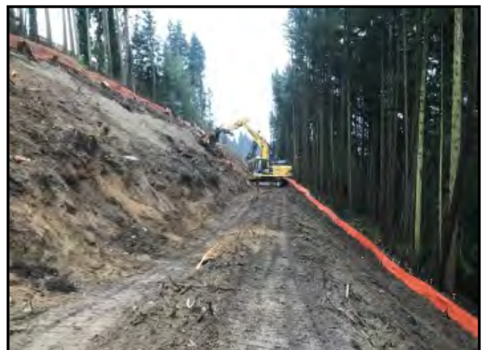
Clearing and grubbing along the temporary access road.
