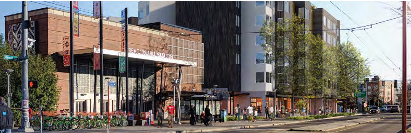
Entrance to the Beacon Hill Station.
