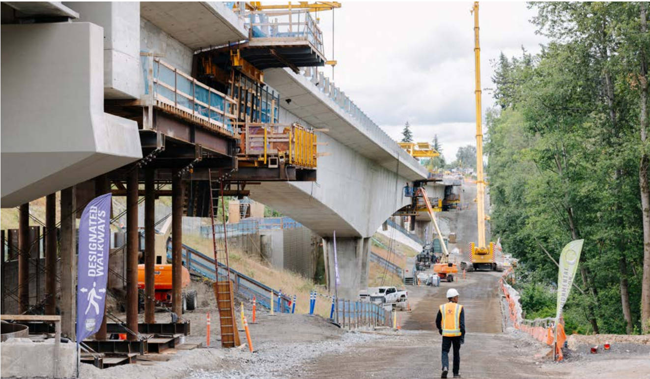
A Sound Transit construction worker examining Structure C, which bridges unstable soil on the Federal Way Link Extension, during a visit on June 2024.
