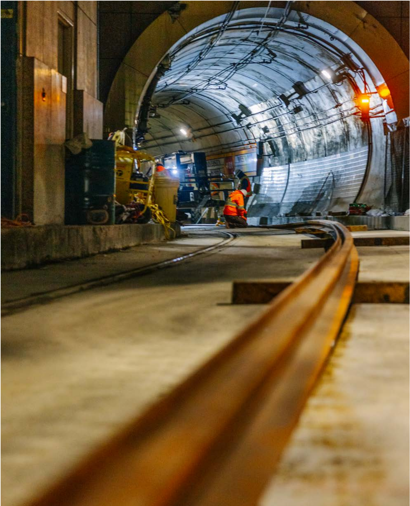
Rail replacement in the Downtown Seattle Transit Tunnel during the service disruption.
