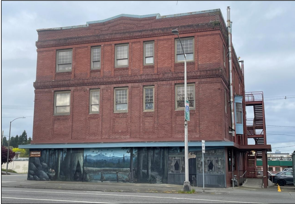
Figure 9-27 View West Southwest, 1515 Pacific Avenue East and North Elevations
