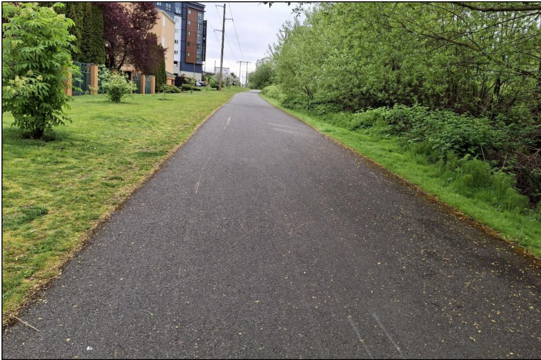
Figure 9-2 View Northeast, Looking Up Interurban Trail From South End of APE
