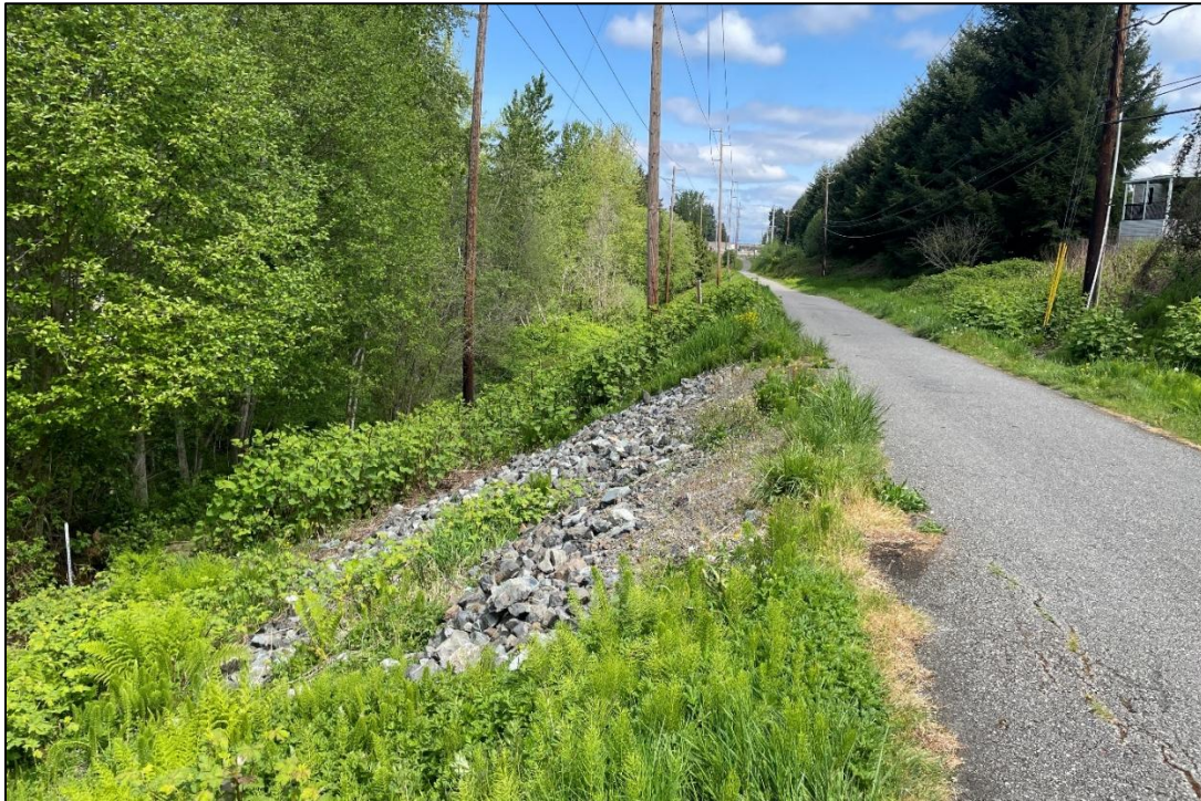
Figure 9-34 View North, Exposed Quarry Spalls, and Cut and Fill Section of Historic Railway Alignment
