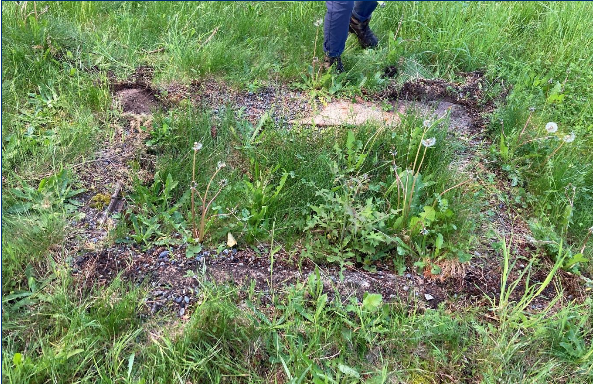
Figure 9-24 View South, Concrete Foundation Covered by Grass
