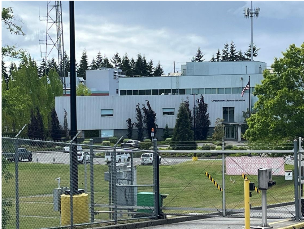
Figure B-EGN-77. Survey Number 222, Snohomish PUD, Building 2, Operations Administration, 1802 75th St SW (DAHP ID Number 734364)
