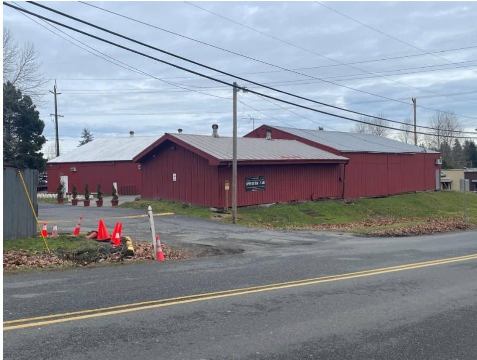
Figure B-AIR-35. Survey Number 137, 11732 Airport Rd (DAHP ID Number 732362)
