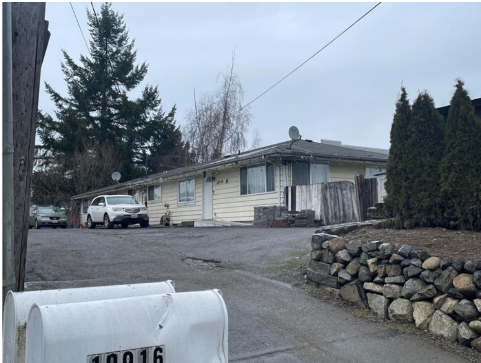
Figure B-OMF Site E-31. Survey Number 697, 10916 Holly Dr (DAHP ID Number 256702)
