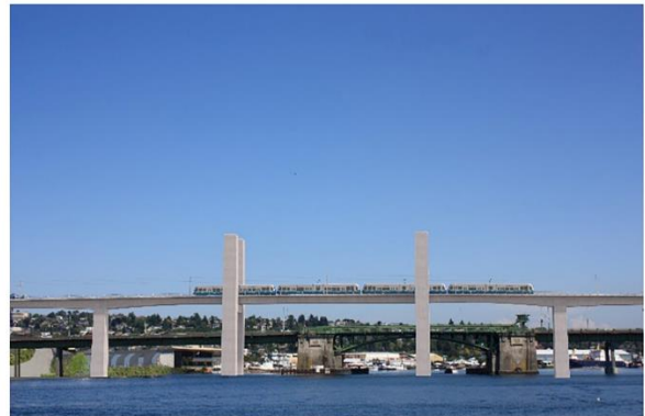
Elevated 15th Avenue Alternative (IBB-3) (vertical lift moveable with balanced cantilever segmental box girder approach bridge type)
