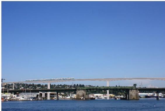
Preferred Elevated 14th Avenue Alternative (IBB-1a) (balanced cantilever segmental box girder bridge type)
