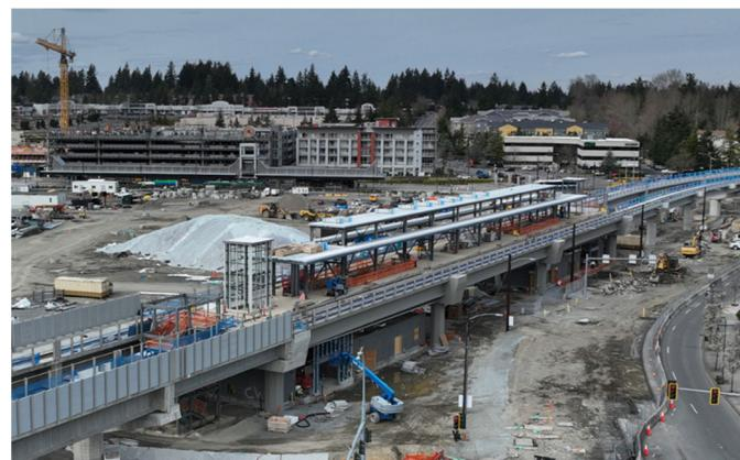
Structural steel and concrete complete at FWD Station
