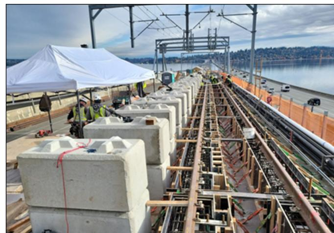
*Formwork in place for plinth pour back at west approach to floating bridge*
