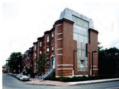
這個波士頓的例子將通風設施與歷史建築結合 This example in Boston illustrates an example of integrating ventilation with historic building
