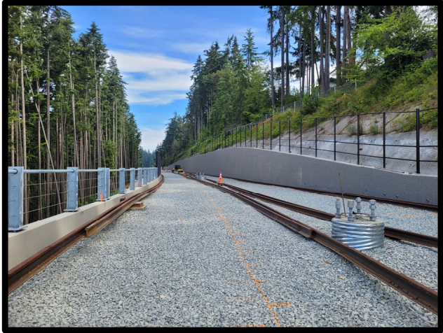
Soil Nail Walls Supporting Guideway in Mountlake Terrace
