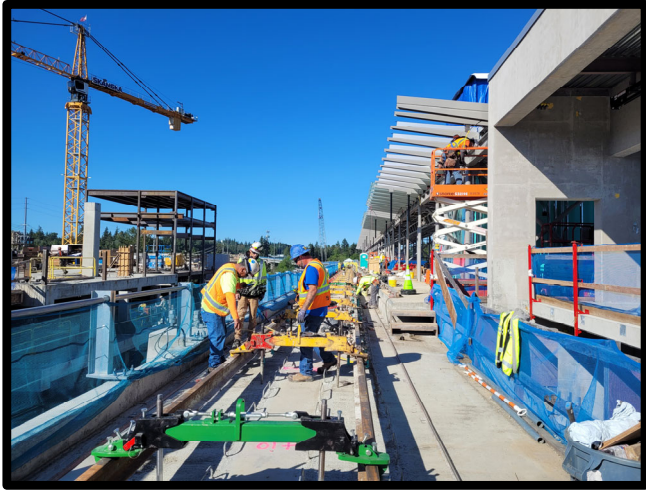
Constructing Track through the Lynnwood Station
