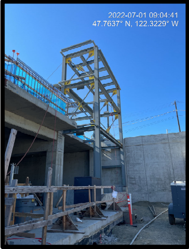
185 th Station Elevator Structure in north Shoreline
