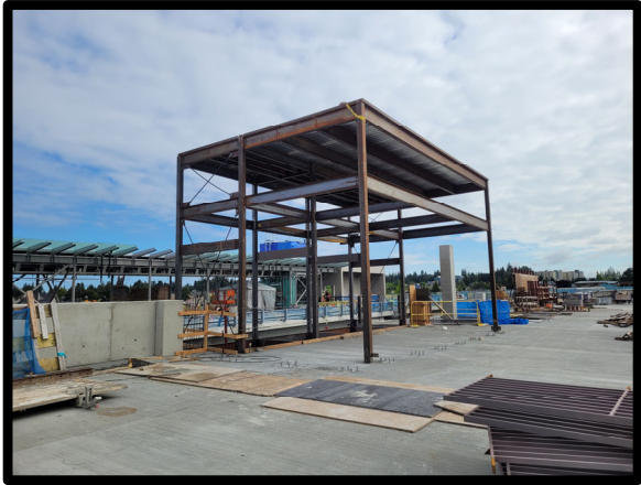
Lynnwood Parking Garage Elevator Structural Steel
