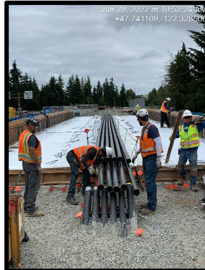
Guideway Conduit Ductbank work in Shoreline
