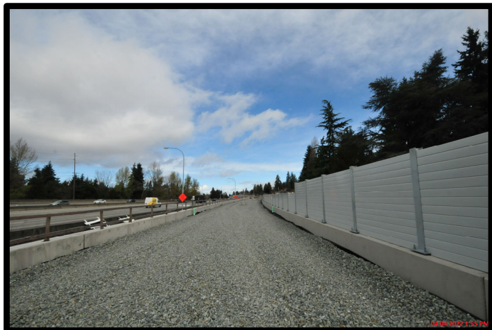
Acoustical Panels Along Guideway in Shoreline
