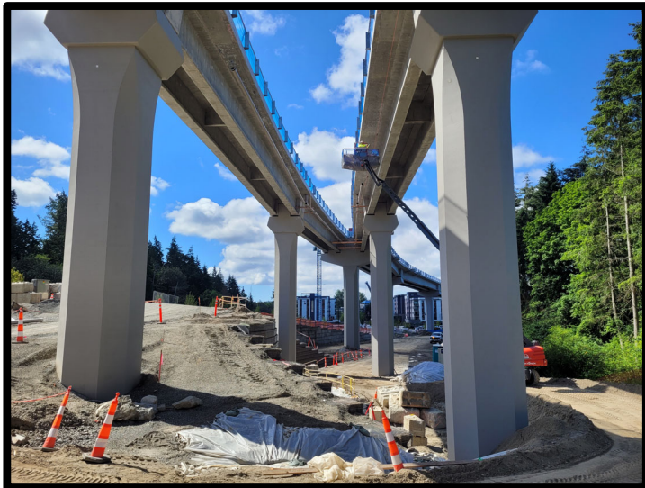
Coating Guideway South of the Mountlake Terrace Transit Center
