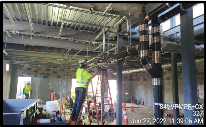
Installing Plumbing and Mechanical in the 148th Station in Shoreline
