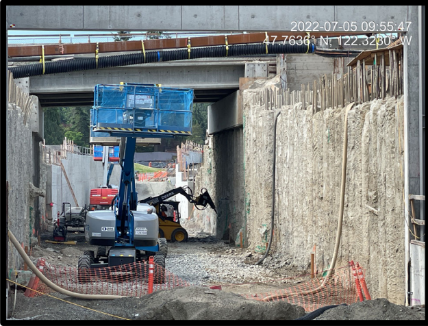
Installation of the Secant Pile Walls for the 185 th Street Undercrossing
