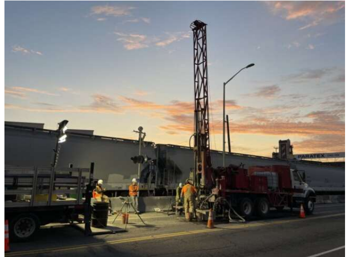
Example of geotechnical drilling equipment
