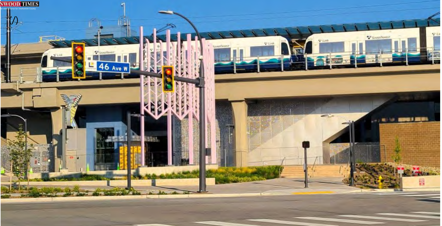
Sound Transit's Lynnwood Link light rail in July of 2024. Lynnwood Times | Mario Lotmore.
