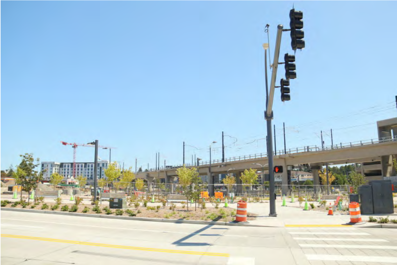
The Lynnwood light rail station during its final weeks of construction. (Photo by Nick Ng)
