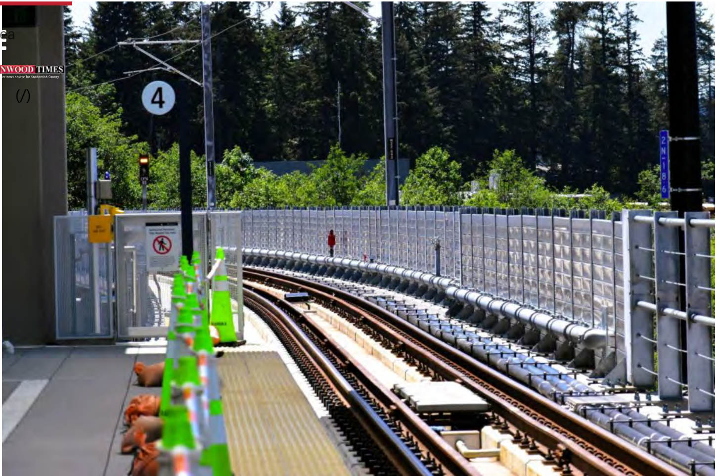
Sound Transit's Lynnwood Link light rail track at its pre-revenue testing, on Friday, June 7, 2024. Lynnwood Times / Mario Lotmore.
