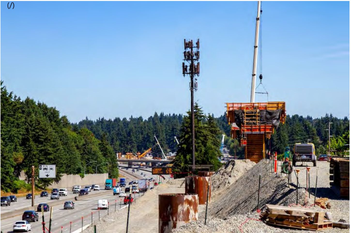
Sound Transit's Lynnwood Link light rail construction at Mountlake Terrace. Lynnwood Times | Mario Lotmore.
