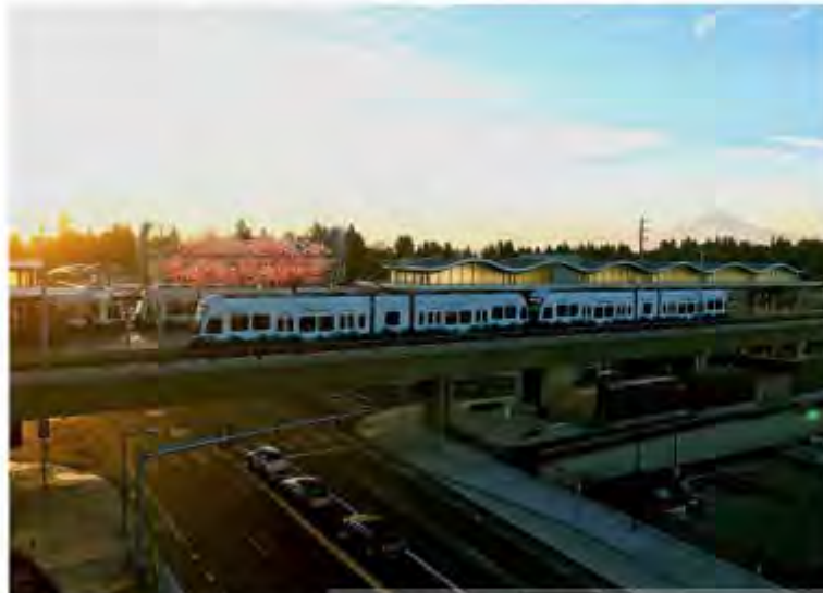
A train departs from the elevated guideway at Angle Lake Station. Elevated guideways allow people to continue biking, walking and driving underneath.
