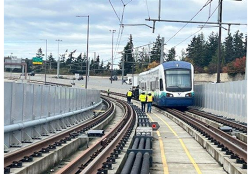
LRV Car Mover and Dead Car Tow Testing East Channel Bridge (Segment 1)
