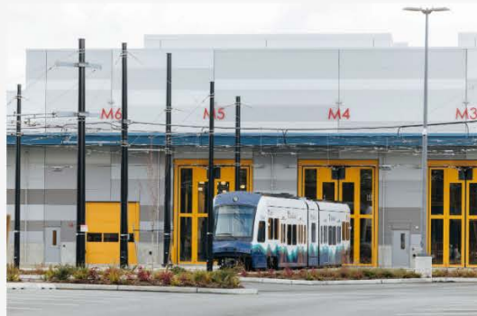
A light rail vehicle sits on the vehicle storage tracks to prepare for regular maintenance at OMF East. | Click on image to enlarge
