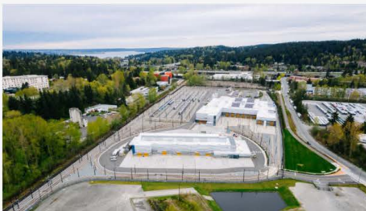
Sound Transit's recently completed 28-acre OMF East property in Bellevue showing light rail vehicle storage tracks and almost 180,000 square feet of various required maintenance shops and other supporting facilities. | Click on image to enlarge
