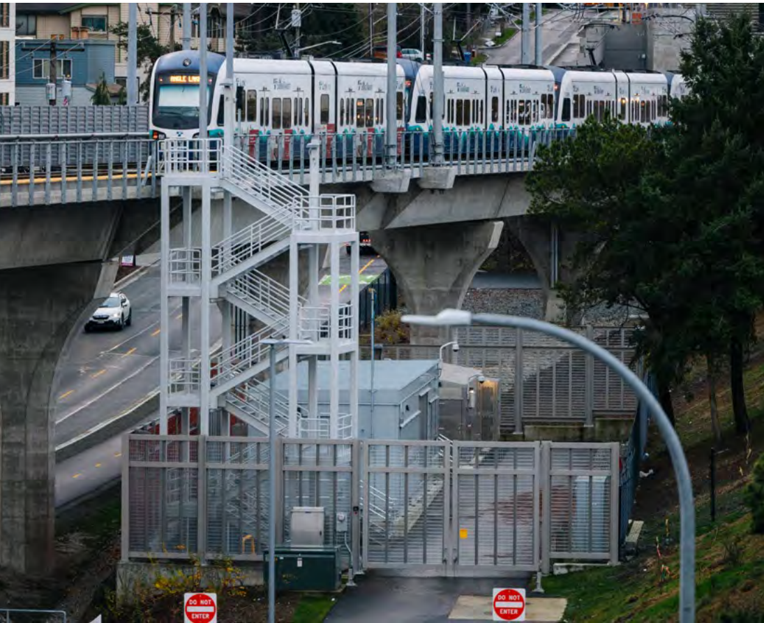
Figure iv for 3.3.12 - Metal grating panels provide screening for the TPSS building at Northgate Station
