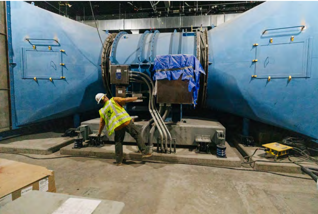
Figure ii for 3.3.12 - Tunnel fan ventilation Room at U-District Station
