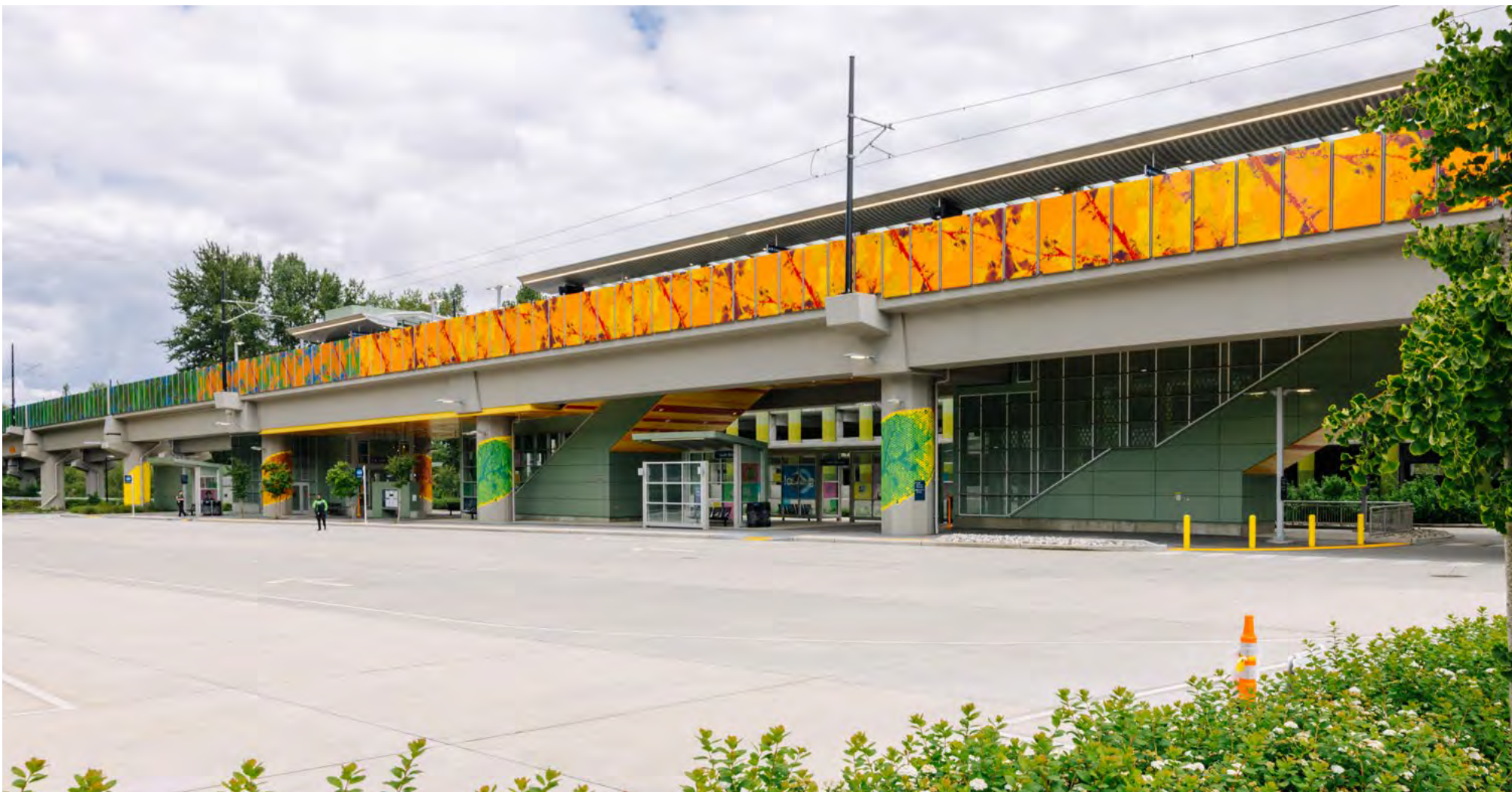
Figure i for 3.2.4 - South Bellevue elevated station with acoustic barriers
