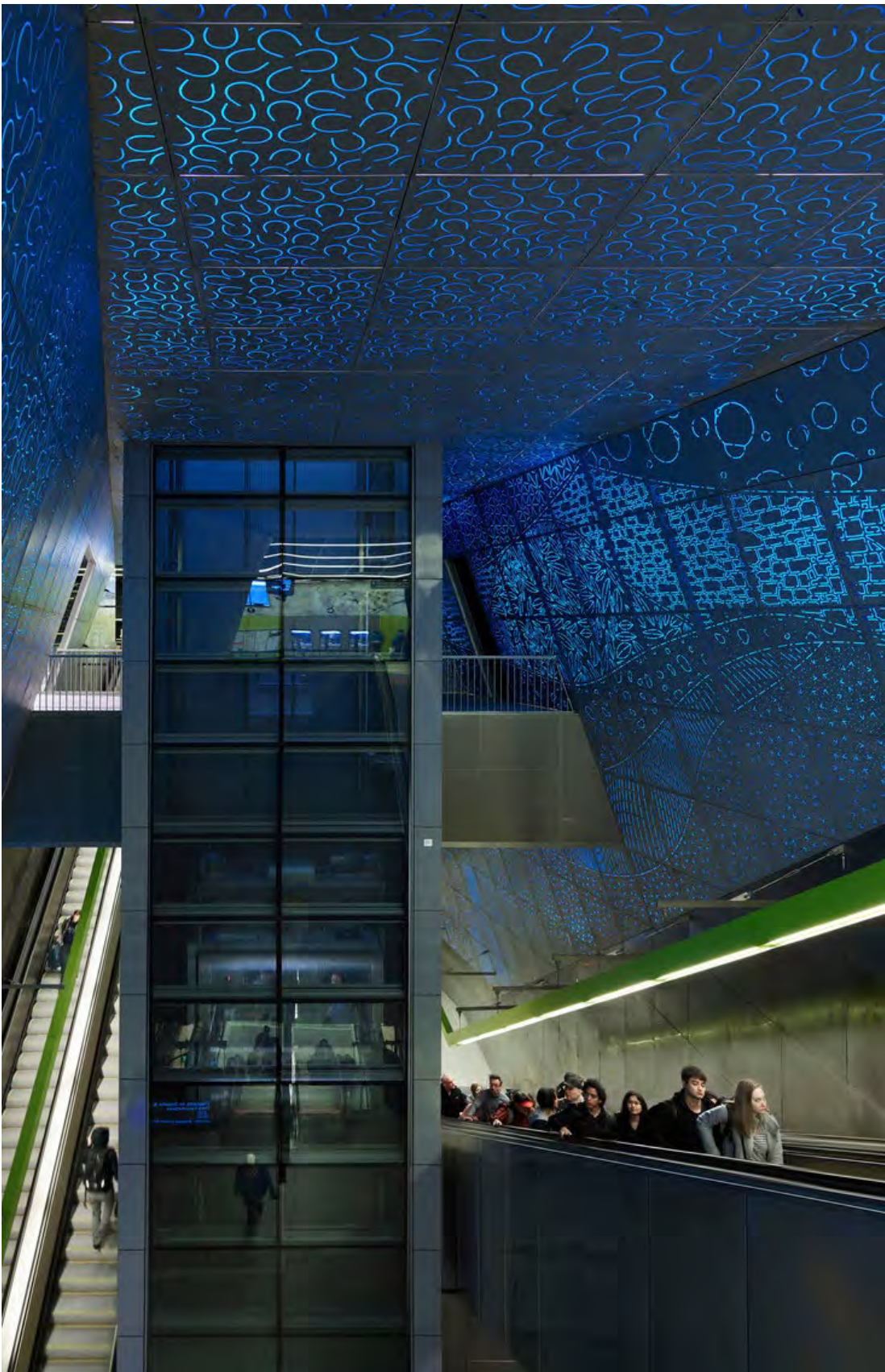
Figure iii for 3.3.6 - Glazed elevator shaft at University of Washington Station
