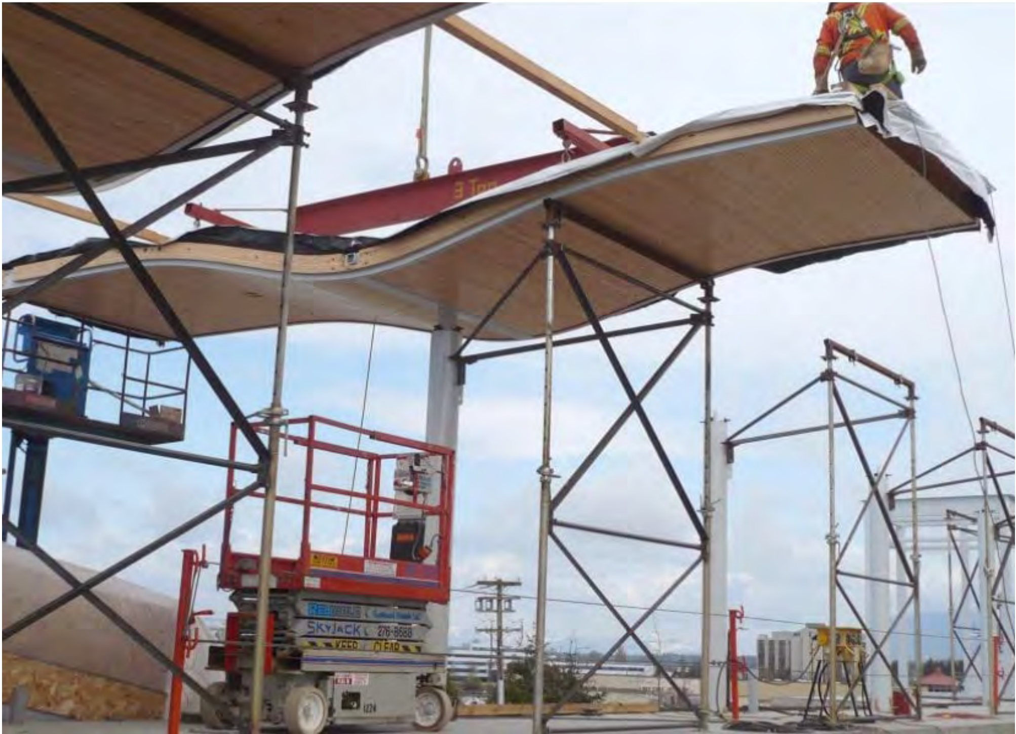
Figure i Hoisting prefabricated elements into place
