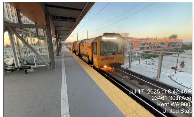
Rail Profile Grinding– Kent Des Moines Station
