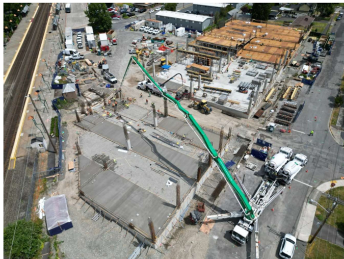
Sumner: Aerial view of concrete Pour 3 and level 2
