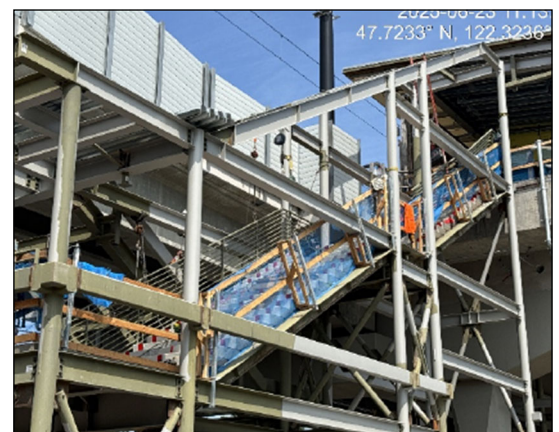
Stairs and guardrail installation
