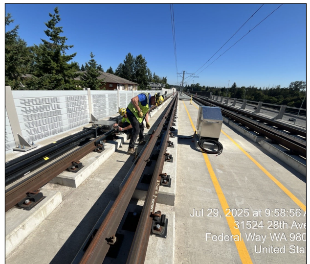
Rail Lubricator Install
