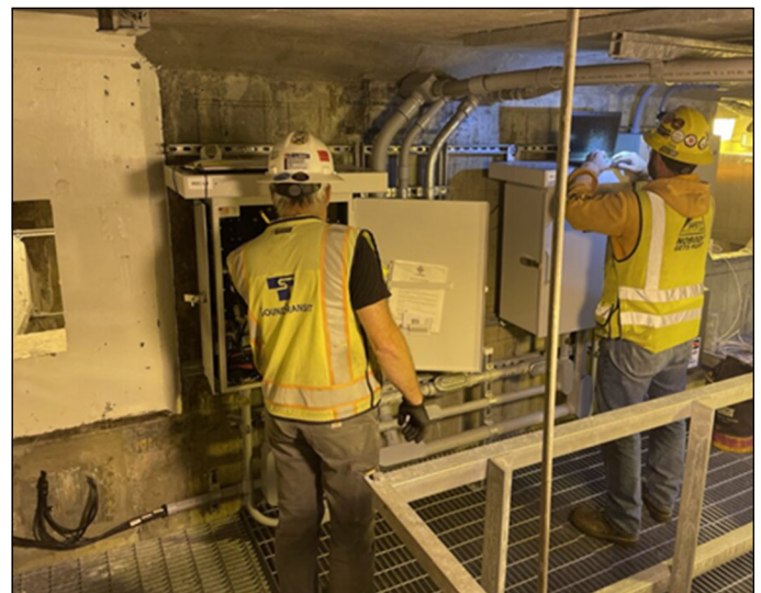
Crews calibrating cathodic protection modules inside floating bridge pontoon
