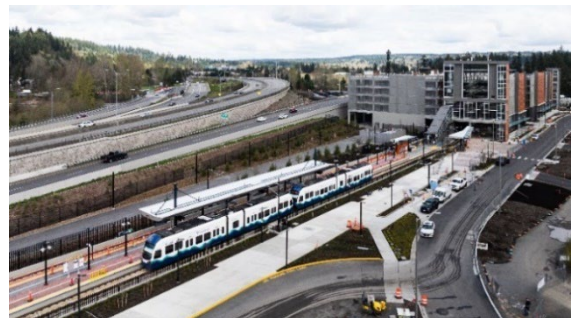
Figure 13: Testing at DRLE Marymoor Village Station during pre-revenue simulated service in April
