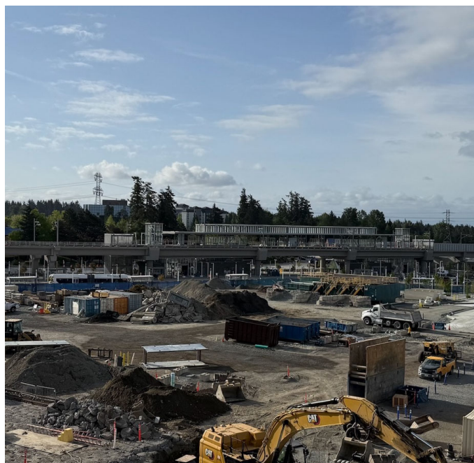
Aerial view of Downtown Federal Way TC construction
