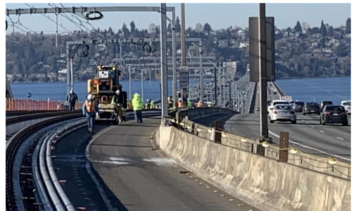
I-90 Signals Installations
