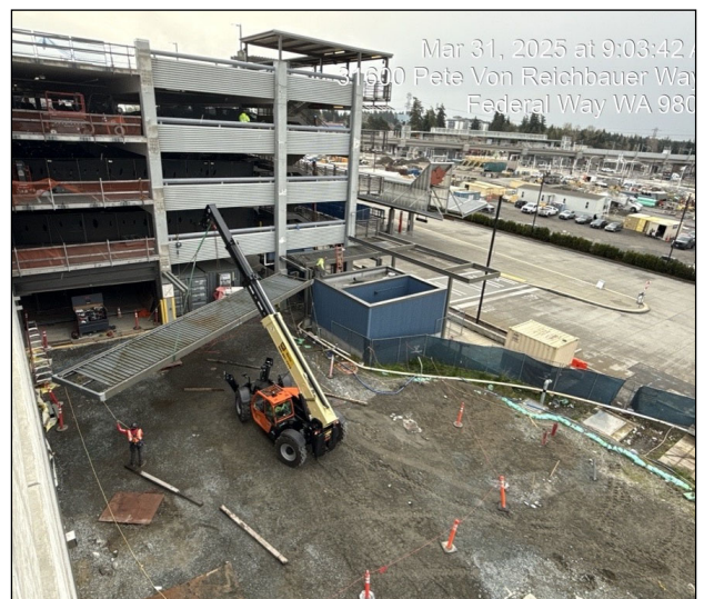
Canopy Install- Federal Way Downtown Garage
