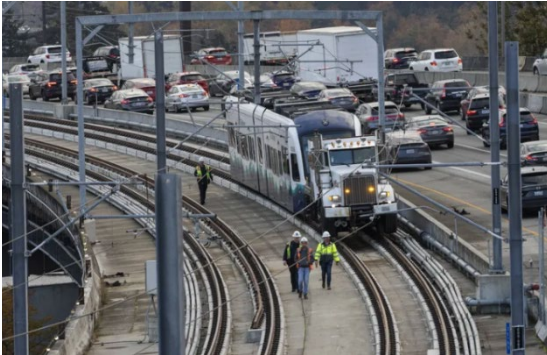
Figure 11: Unpowered LRV Clearance Tow Test across the East Channel Bridge in April
