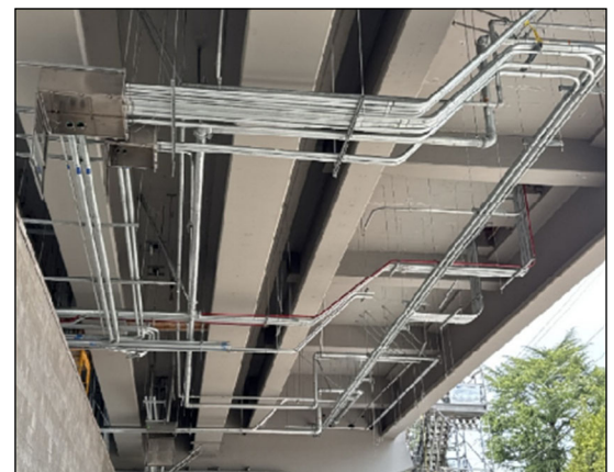
Under guideway conduit installation
