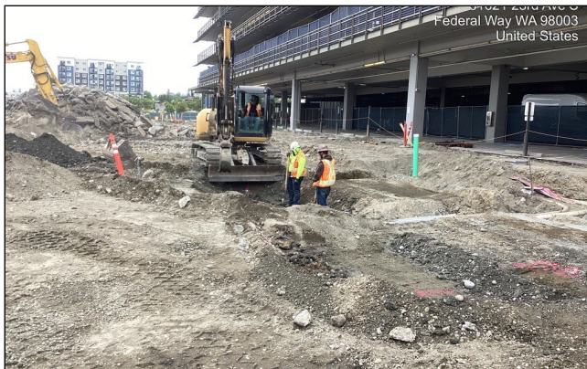
317th Str. Water Service Tie-in Installation
