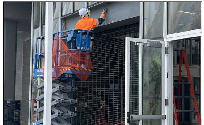
Structural Steel Painting– Kent Des Moines Station
