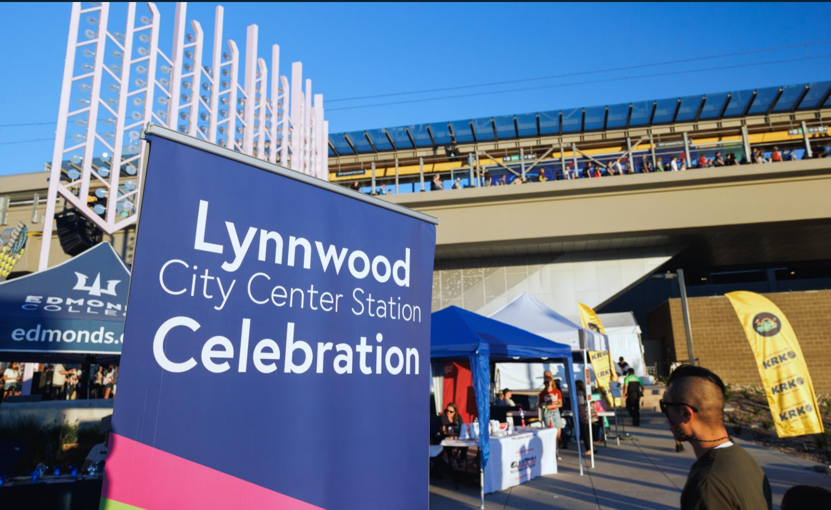
With the Lynnwood Link Extension now open, land adjacent to the Lynnwood City Center Station that was needed during construction is set to become affordable housing.
