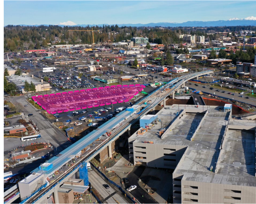
Lynnwood City Center construction with TOD site (in pink)
