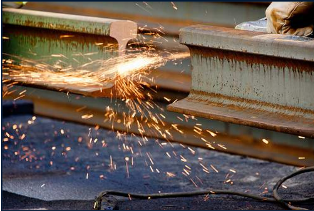
Capitol Hill Station Rail Construction
