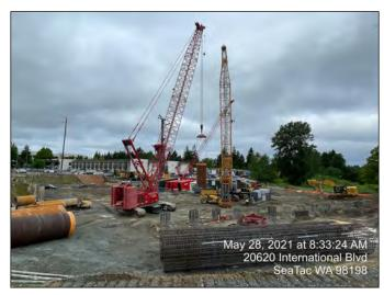
Installing slip casings for Pier 2 at SR-99 Bridge (SW)
