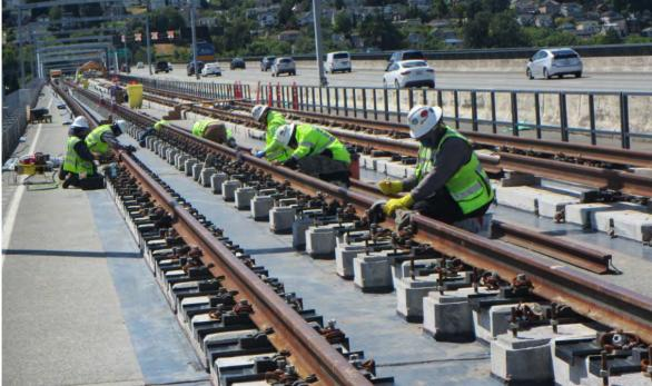
E130 Seattle to South Bellevue: Removing wax tape along the I-90 east bound track way
