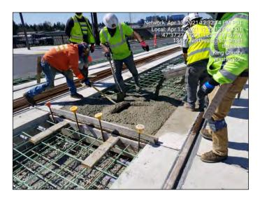
Placing concrete in the center track slab facing west.
