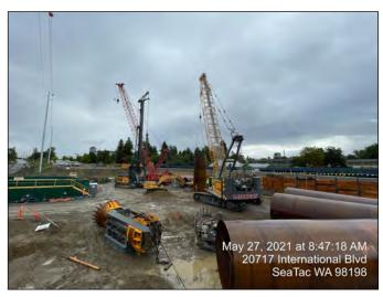
Setting foundation casings at SR-99 Bridge (NE)
