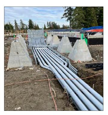
Signal house foundation and conduit placement
