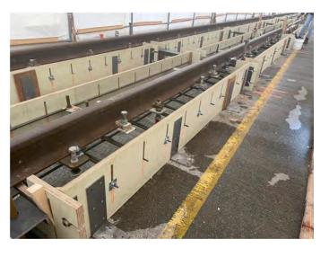
Formwork in place for plinth construction mock up
