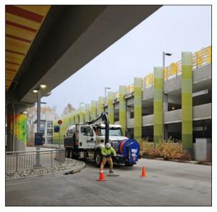
Contractor performing storm sewer jetting to remove line-blocking debris at South Bellevue Station
