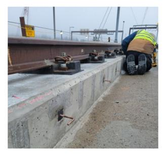
Crews weld stray current studs on D2 roadway plinths
