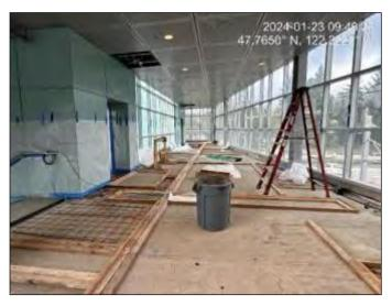
185th station pedestrian overcrossing concrete formwork
