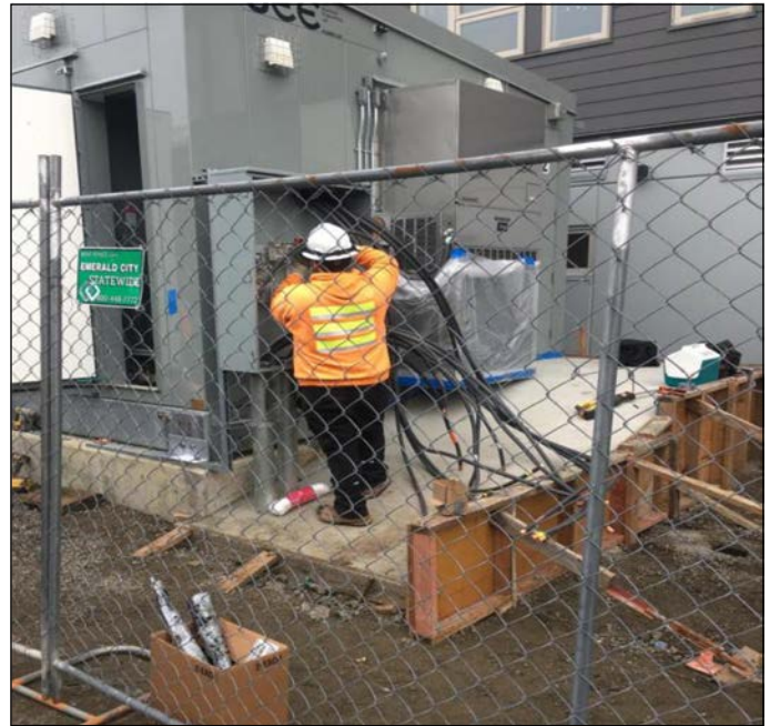
Landing TPSS #4 power wires– H3
