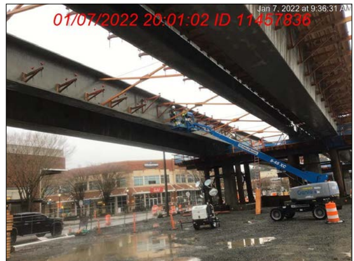
Working on girder brackets and cross bracing at Downtown Redmond Station.
