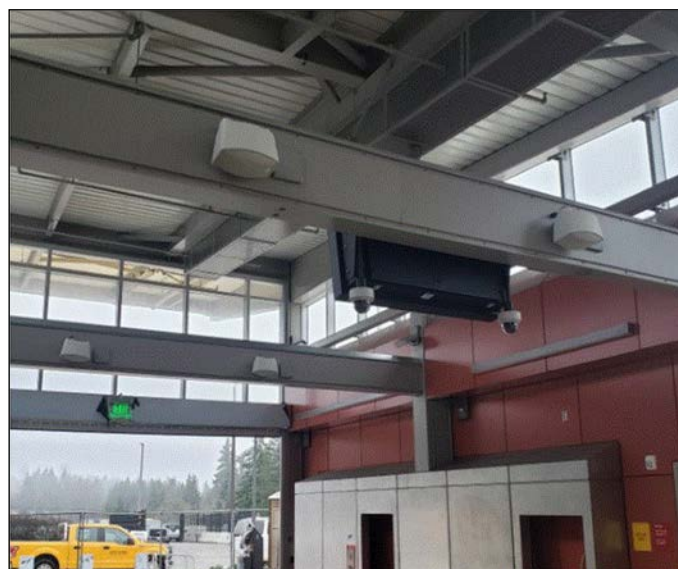
Installation of PA equipment at Mercer Island Station.
