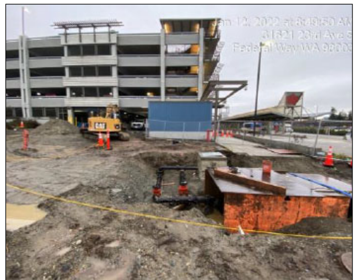
WA3.8 Waterline Installation at Federal Way Transit Center
