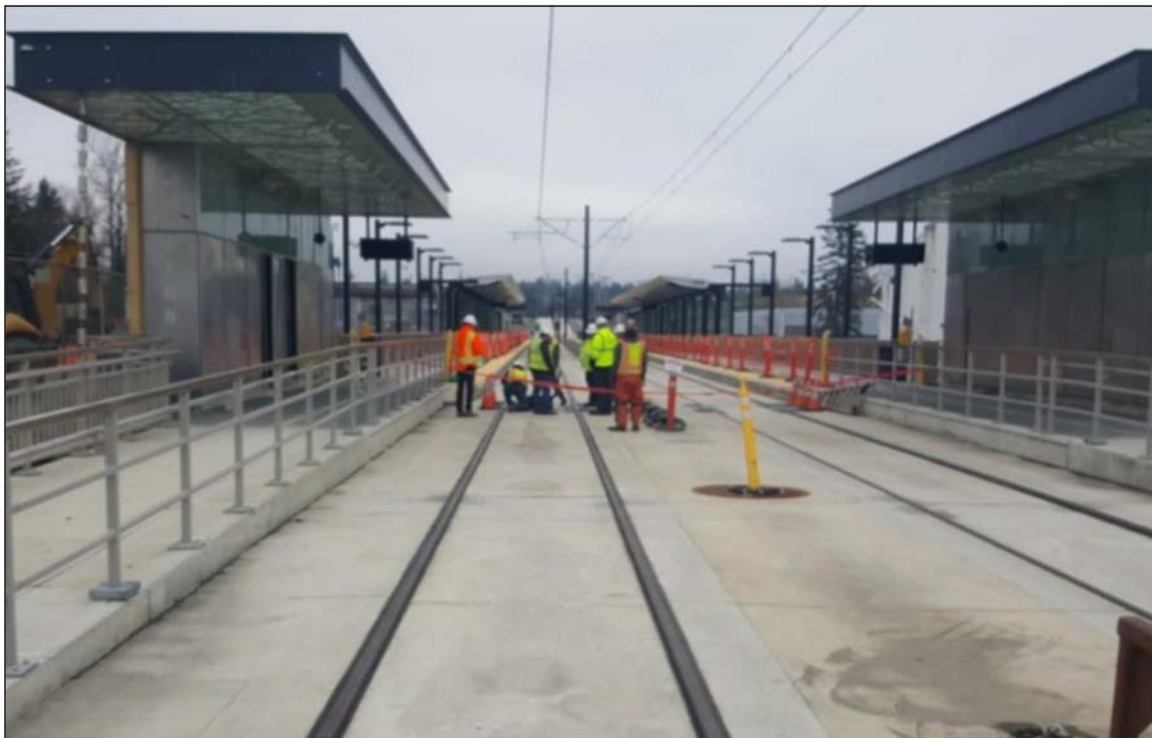
E340 Bel-Red: E340 Contractor conducting Rail to Earth testing on the embedded track section at the 130th St Station .
