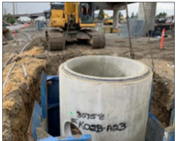
WA1.3 Installing Storm Drain Str.
