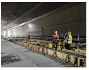
Survey crews check alignment of formwork installed for plinth rebuild in Mount Baker Tunnel
