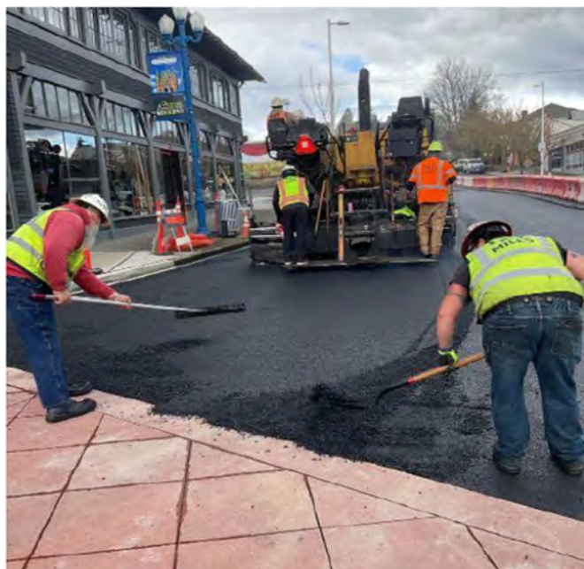
Paving North I Street
