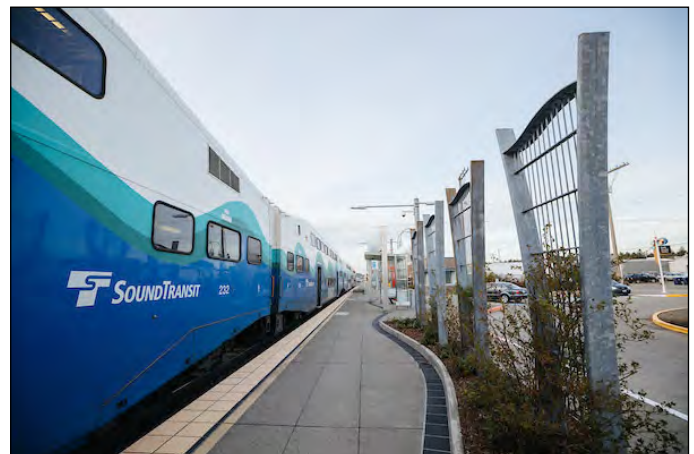
South Tacoma Station Passenger Platform Access
