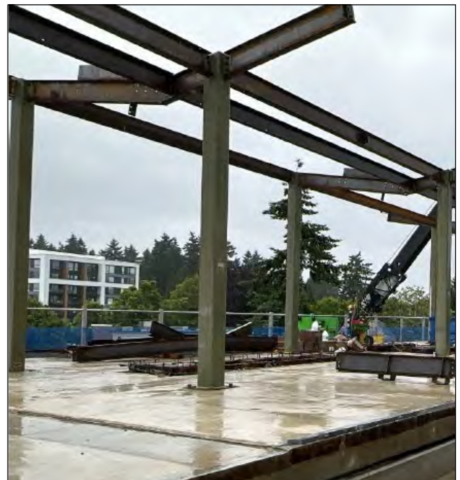
Steel Erection at Downtown Redmond Station Platform
