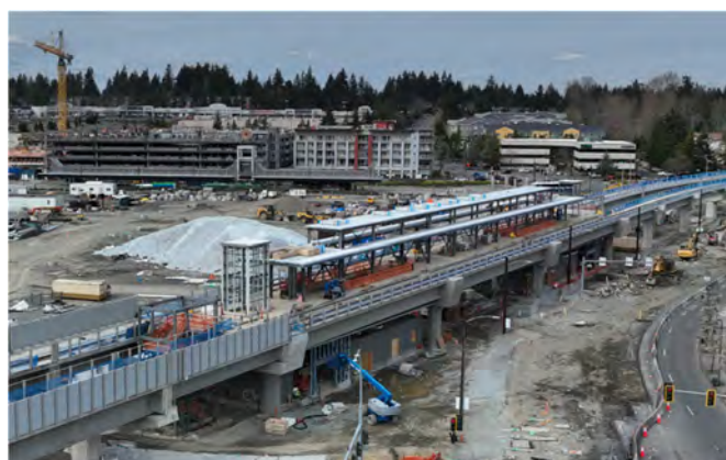
Structural steel and concrete complete at FW Station
