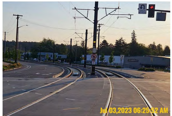
Street level track at Spring Street looking east
