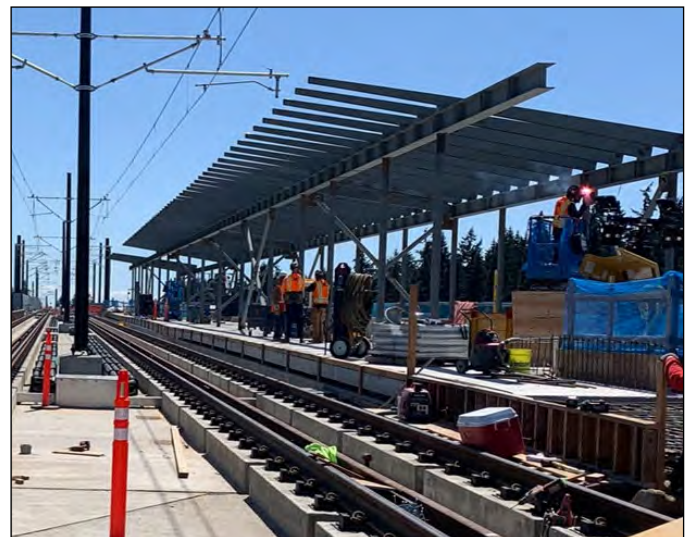
Canopy steel installation
