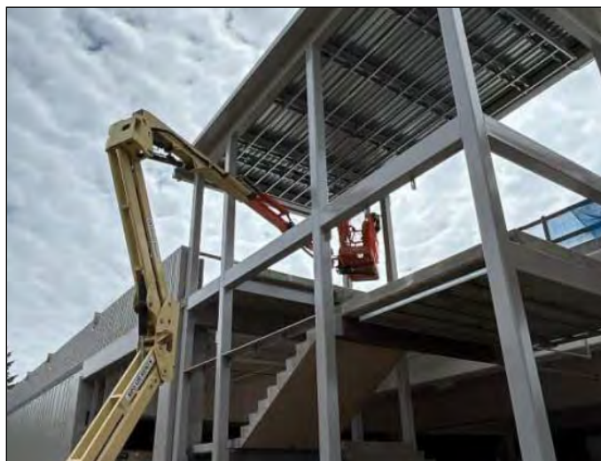
185th St. garage stairwell lighting conduit installation
