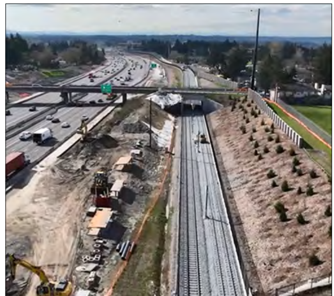
Ballasted track and traction power pole installation started
