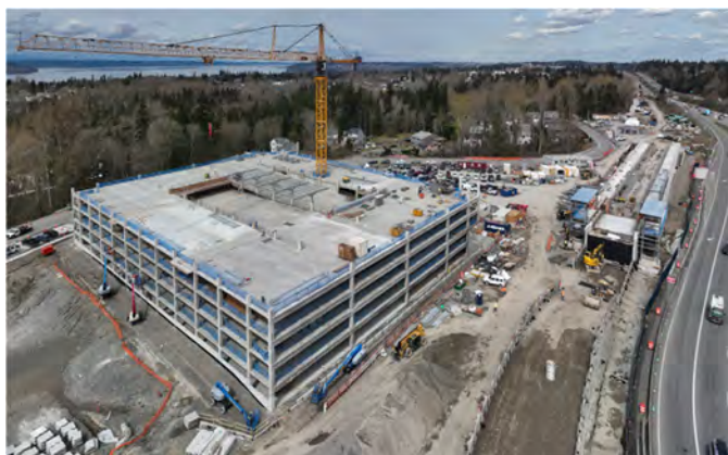
Station finishes underway at Star Lake Station and Garage
