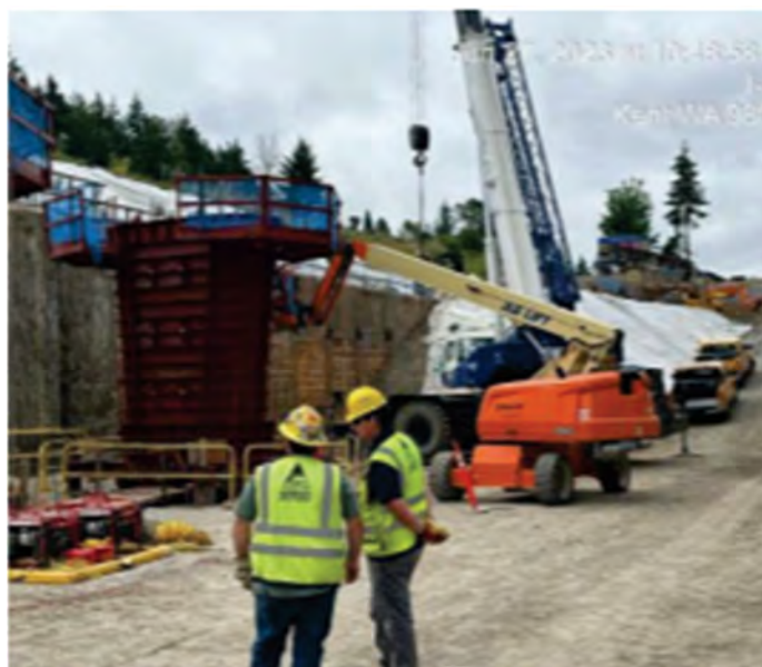
Structure C C06B Column Form in Kent
