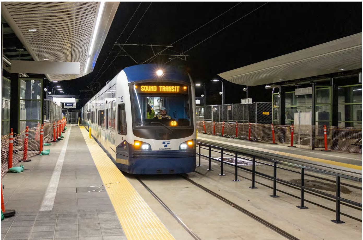
Live wire testing of LRV in the Bellevue segment of East Link
