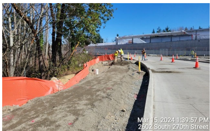
270th W Sidewalk Grading
