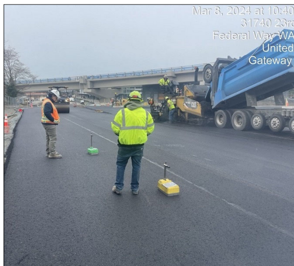
Bus Layover Second Lift Hot Mix Asphalt
