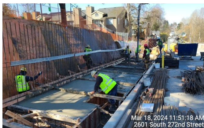
Wall R37 Footing Concrete Placement
