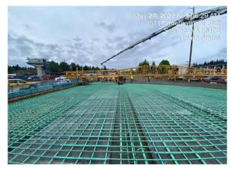
WA 1.1 Kiewit SR99 Span 2 Deck Concrete Placement
