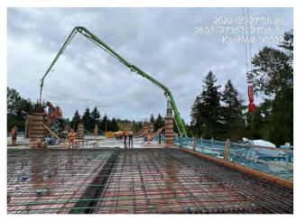
WA 2.4 SL Garage Column Concrete Placement at P3
