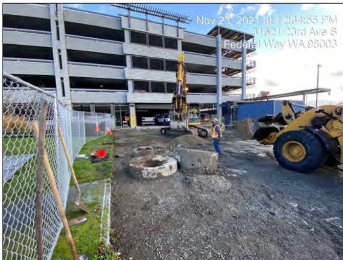
WA 3.8 FWTC Storm Sewer Excavation
