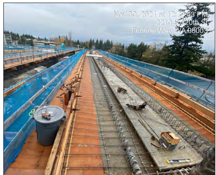
WA3.8 Guideway Deck Reinforcement at Span G20L
