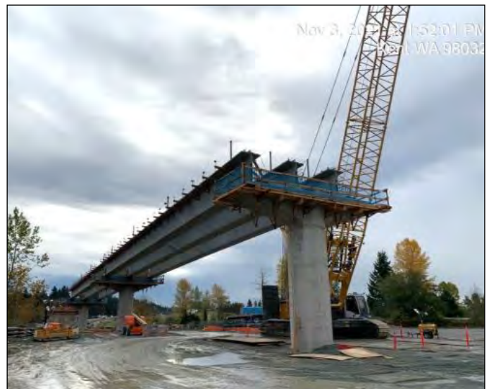
WA3.3 Span 29 30 Erected Overnight
