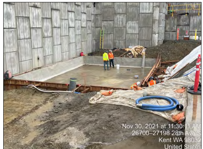
WA 2.4 SL Garage Waterproofing for Elevator Foundations
