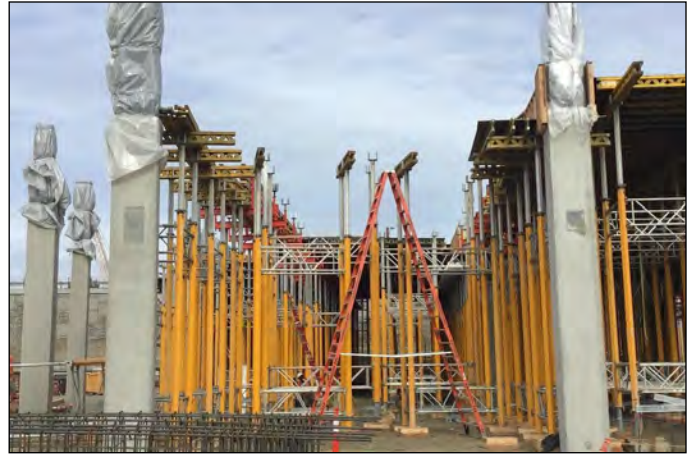
Parking garage deck formwork.
