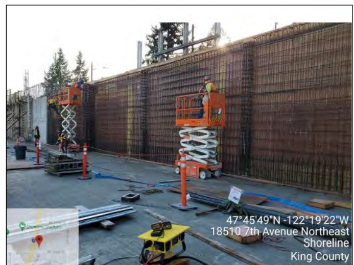
185th garage south wall rebar installation
