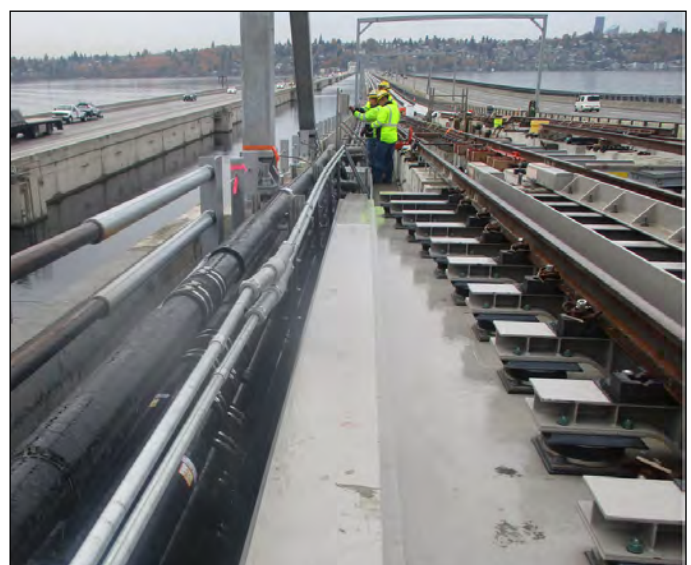
Crews install rigid conduit expansion joints along the above ground ductbank, east approach to floating bridge
