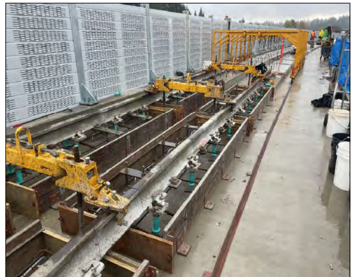
Trackwork and plinth installation.
