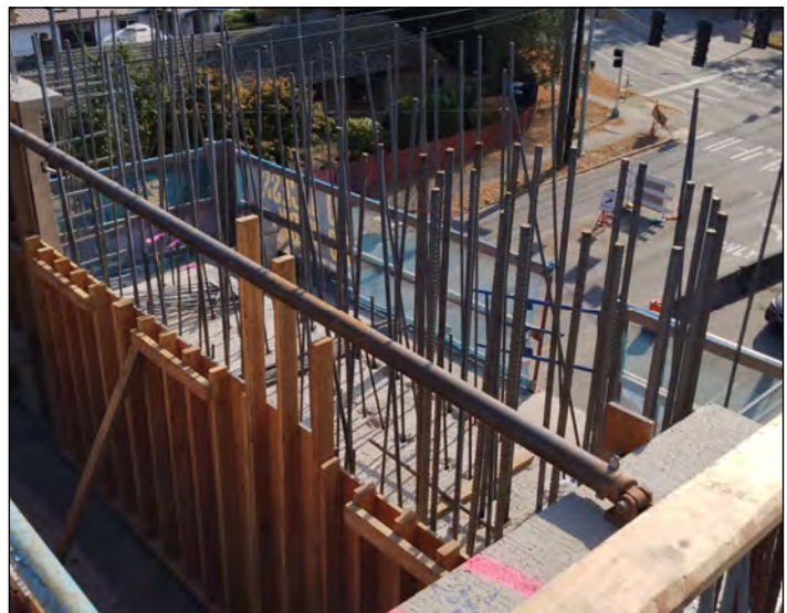
End Diaphragm rebar
