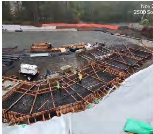
WA2.4 Star Lake Station Footing Rebar Placement
