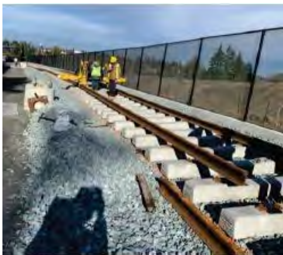
WA1.2 Installing Rail on Ties
