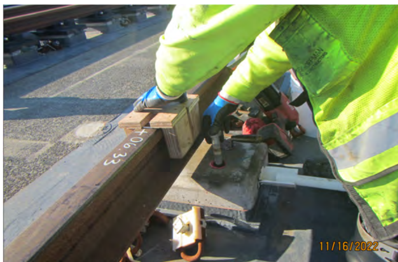
E130 Seattle to South Bellevue: Installing new nylon inserts, westbound on the floating bridge.
