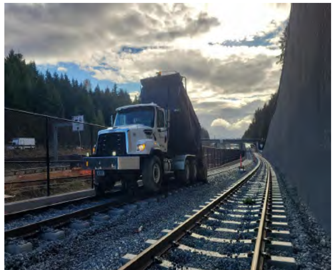
Placing Ballast North of Mountlake Terrace
