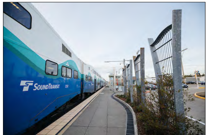
South Tacoma Station Passenger Platform Access
