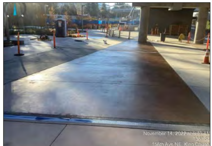
Sealed Decorative Pavement at RTS South Side Plaza
