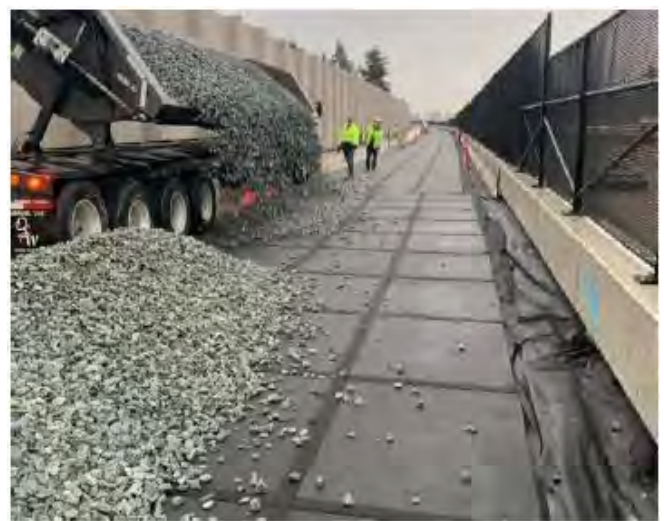
WA1.2 Grading Ballast 1087
