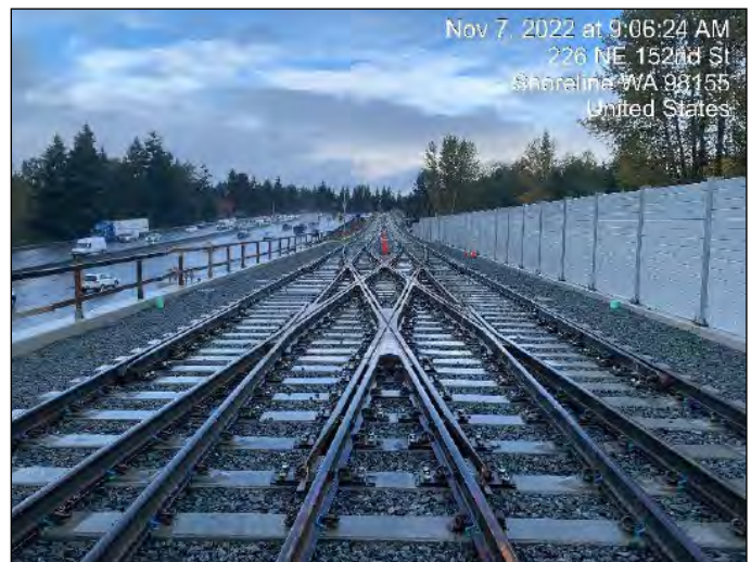
Ballasted track installation
