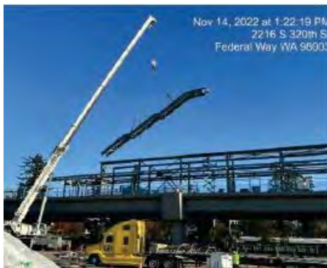
WA3.8 FWD Steel Stair Installation
