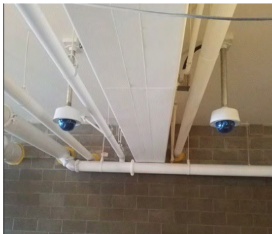
Installation of security cameras at parking garages
