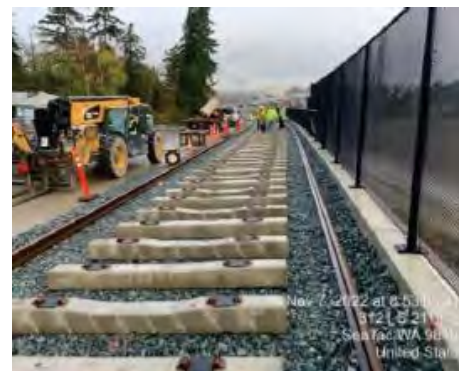
WA1.2 Concrete Tie Placement
