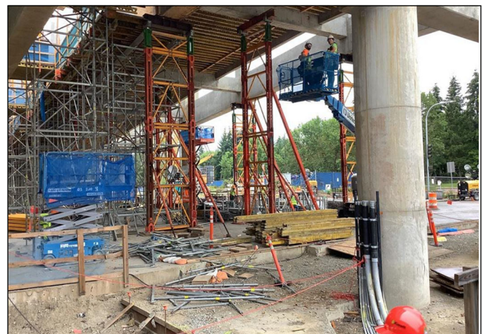
Shoring Removal at RTS Garage Rebuild
