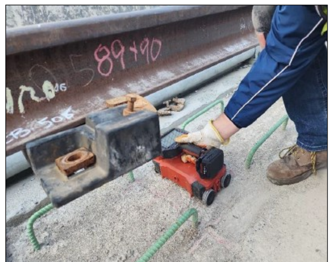
Conducting GPR scanning to locate steel reinforcement prior to plinth reconstruction
