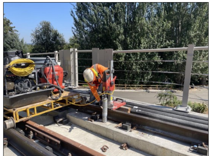
Crews Coring Plinths for Fastener Insert Re-installation
