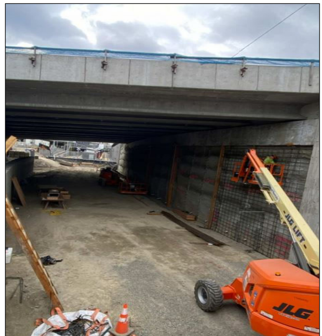
Install CIP Walls at 40th Street - Cut and Cover.
