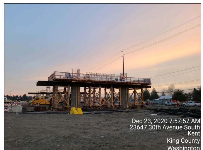
Reinforcement placement at Column B13 cap
