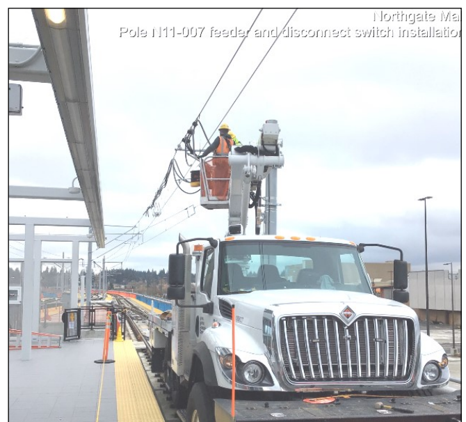
Feeder and disconnect switch installation at Northgate Station.
