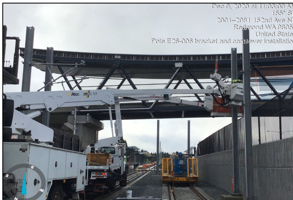
E750 Systems: OCS Pole installation along E360 SR520 to Redmond Technology Station segment.
