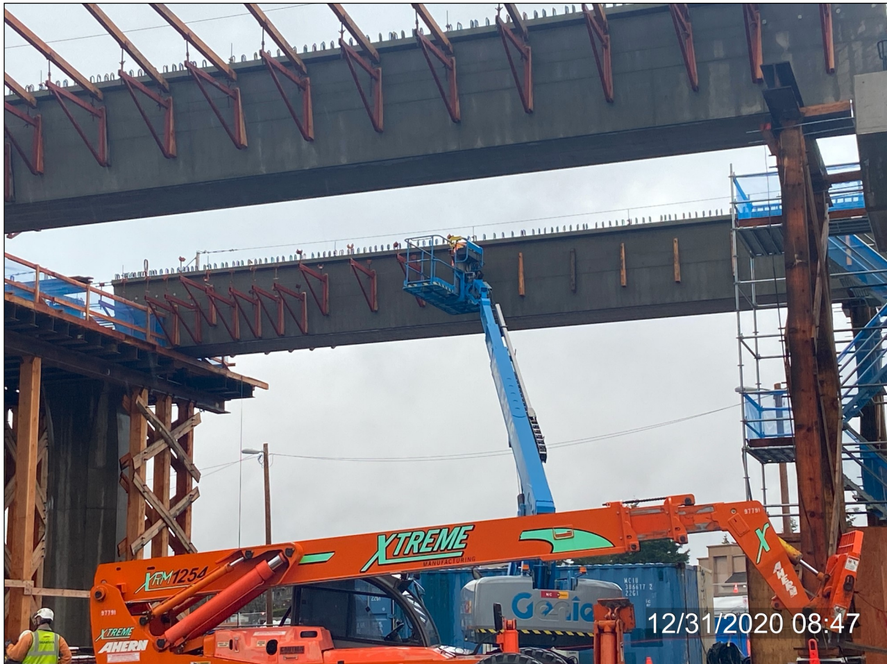
Overhang Brackets Installation (Lynnwood Link Extension)
