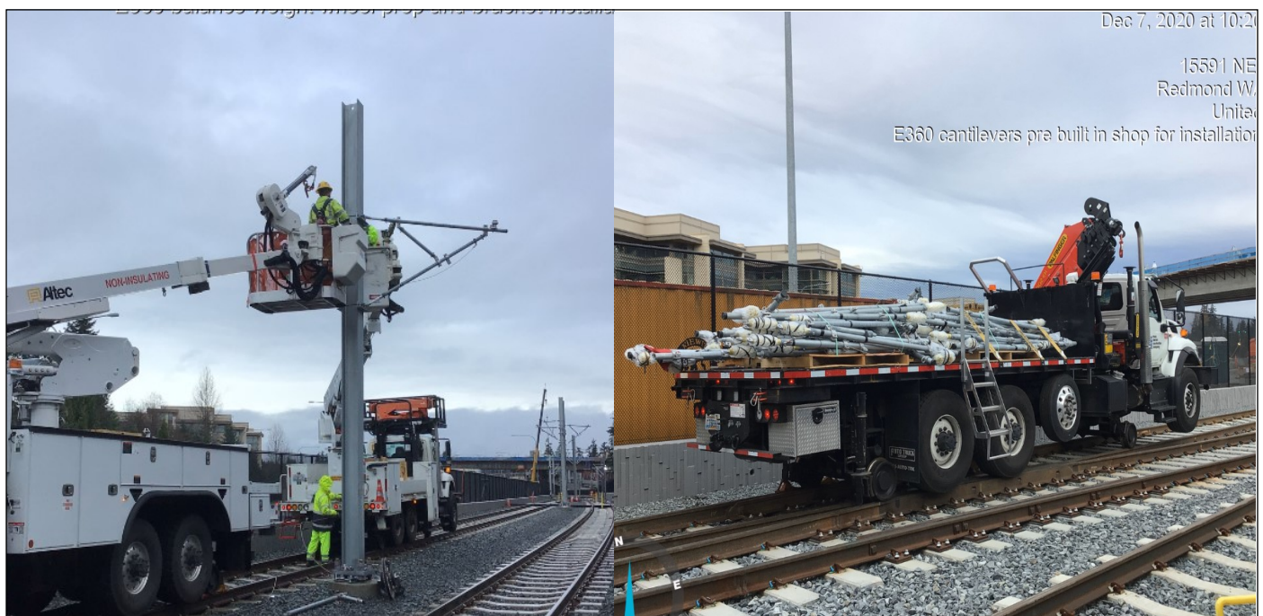
E750 Systems: OCS cantilever installations along E360 SR 520 to Redmond Technology Station segment.
