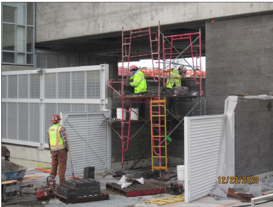
N160—Workers completing section of CMU block masonry wall at Northgate Station.
