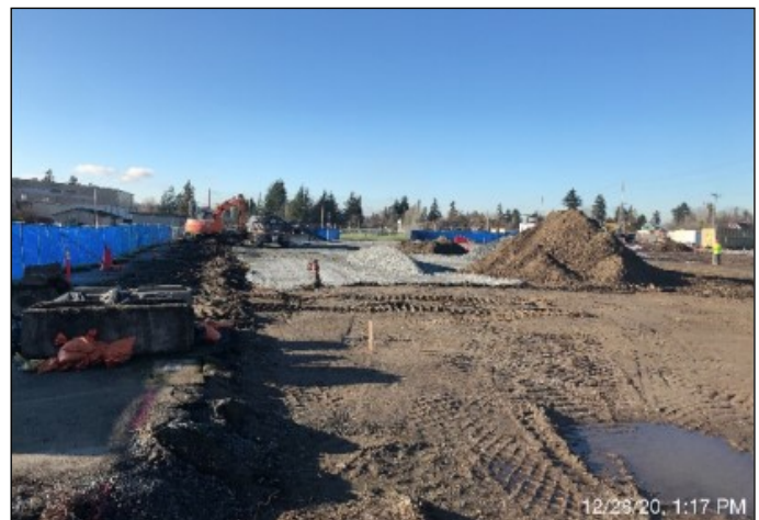
Grading for stone columns installation in garage area.
