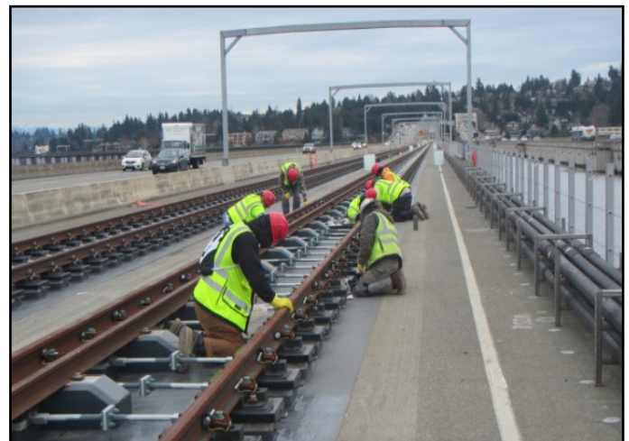
Crews remove wax tape from track tie-down bolt inserts on floating bridge plinths.
