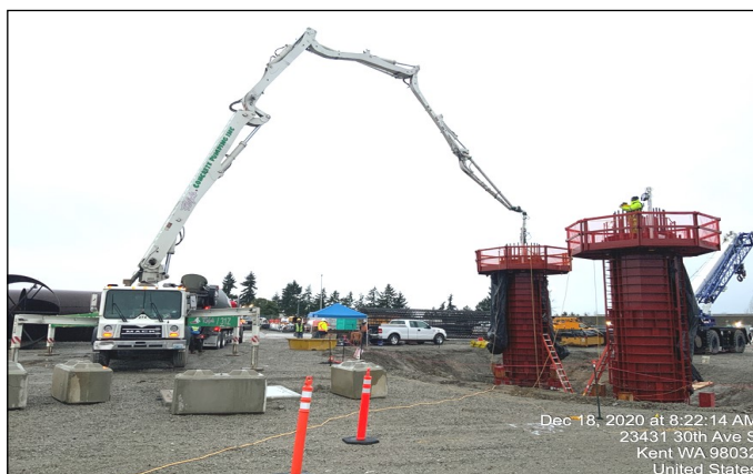
Column and concrete placement
