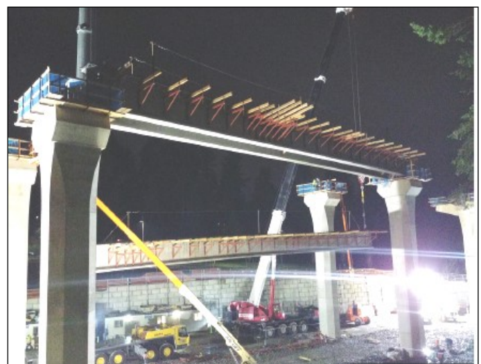
Setting girders at span F31-F32.
