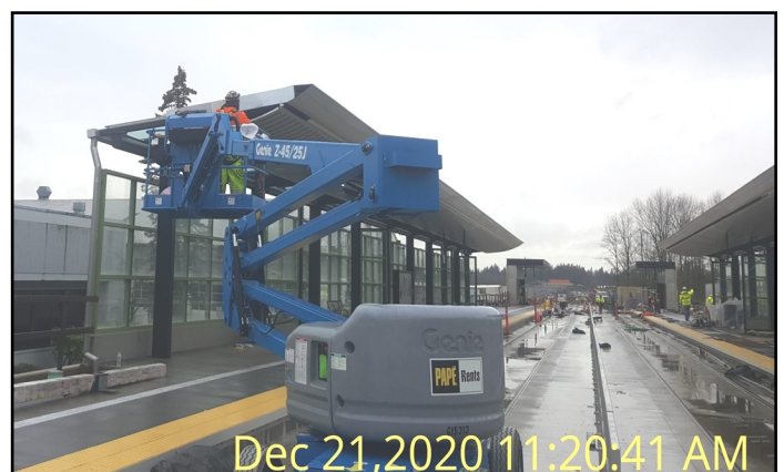
Skirt and end cap installed at south side platform canopy facing west .
