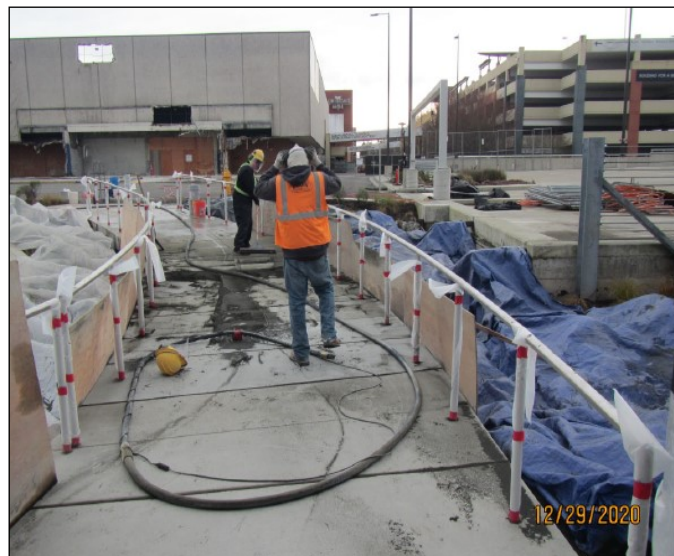
N160—Workers sandblasting the pedestrian bridge over the raingarden at Northgate Station.
