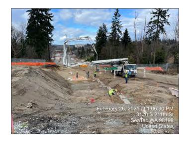
MSE Wall 1018 (NW) Leveling Pad Concrete Placement
