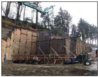
WA08 - Placing concrete at abutment wall G01 footing.
