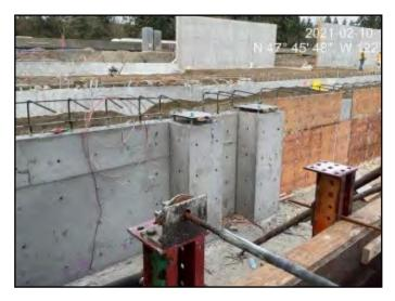
185th station platform wall formwork removal.
