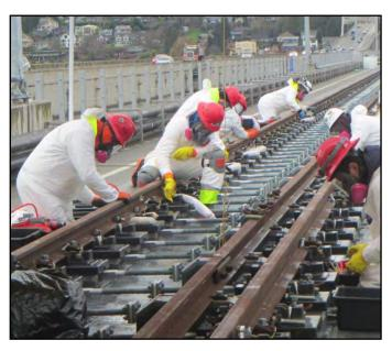
Crews remove wax tape from track attachments on floating bridge
