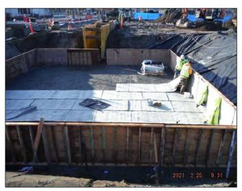
Waterproofing installation at elevator pit.
