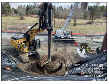
Drilling for B23 foundation casing E at WA2.1
