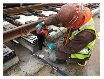
Picture showing the correct drilling depth for reinforcing steel looing southwest.
