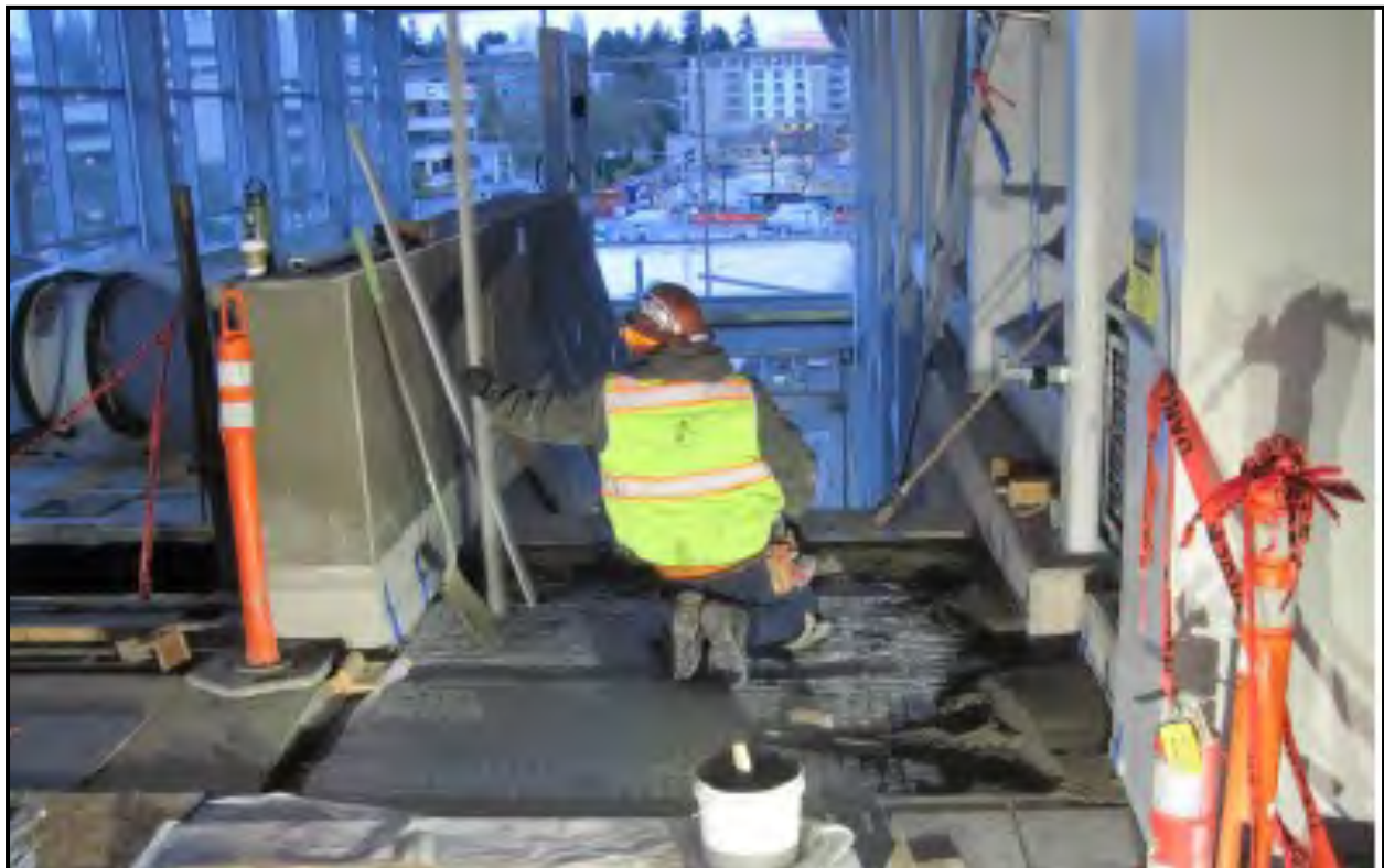
N160 – Western Tile Mezzanine Stair 3 Setting Grout
