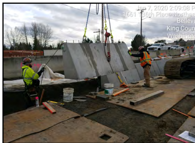
Setting track walls at E340.
