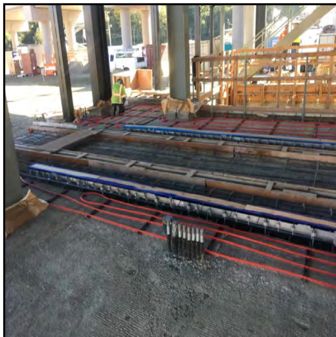
Floor Slab Preparation—OMF
