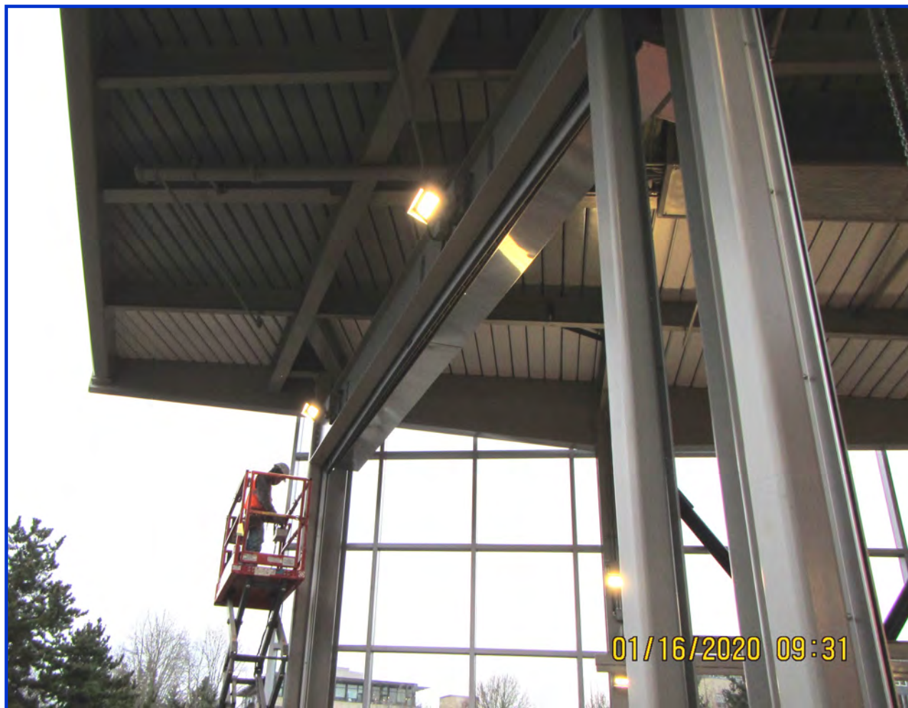
Metal Framing Installation at the Mercer Island Station
