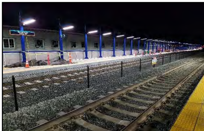
Possible platform and track improvements
