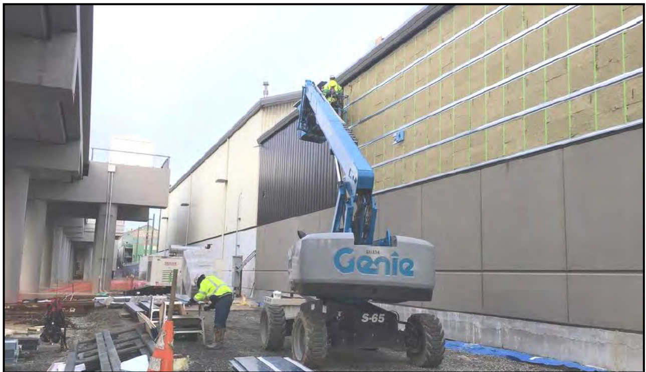
Installation of exterior panels at south side of OMF
