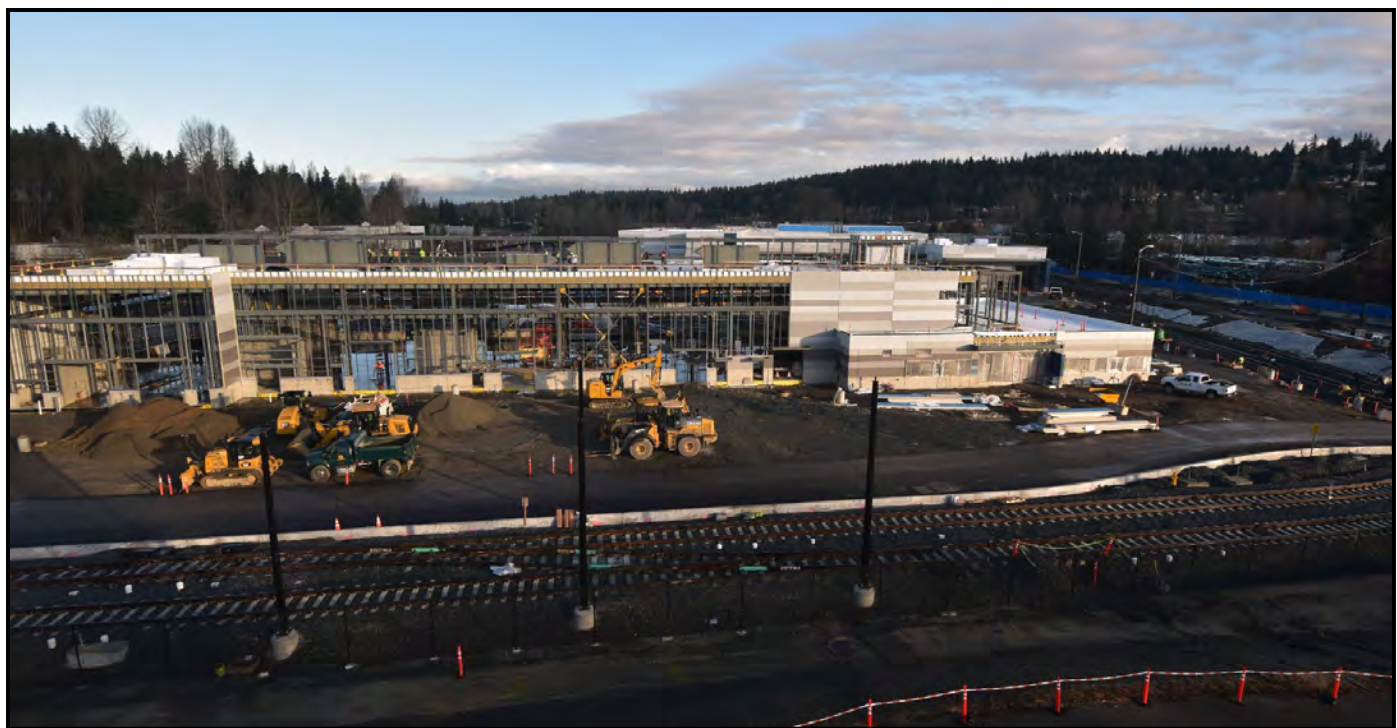
OMF East birds eye view looking north taking shape with yard scope and steel structure framing
