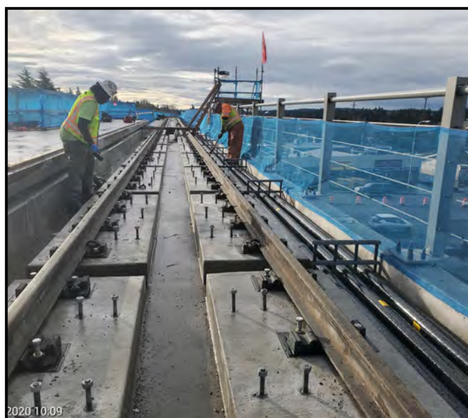
Track work, clipping and alignment at Hospital path.
