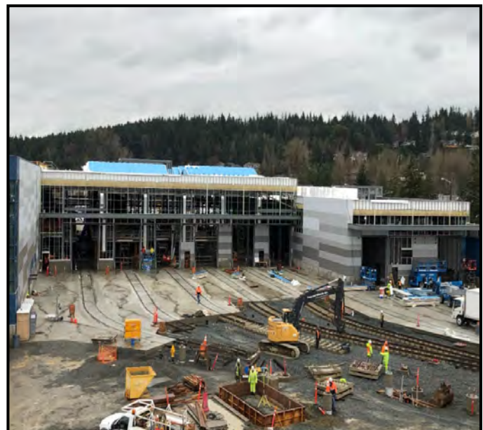
OMFE—Building panel and south apron track installation
