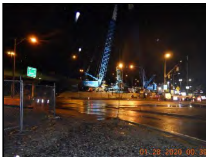
WZ-1 drilled shaft A9
