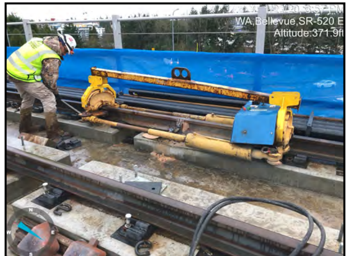
Work Area 2 Aerial Guideway — De-stressing tracks along SR 520.
