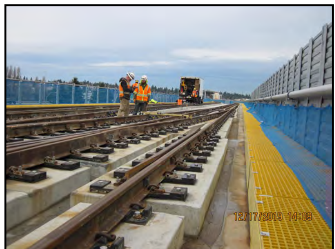
Punchlist work on elevated guideway.
