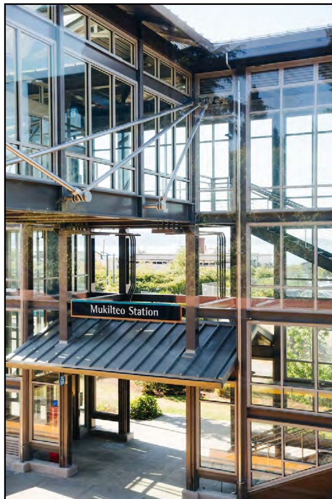
Sounder Mukilteo Station Access Improvements
