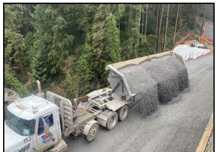
Placing crushed base for WA-1 temporary access road.
