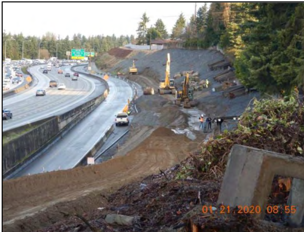
Grading and building eco block wall by I-5 south for L200
