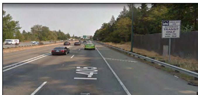
Examples of Bus-on-Shoulder facilities
