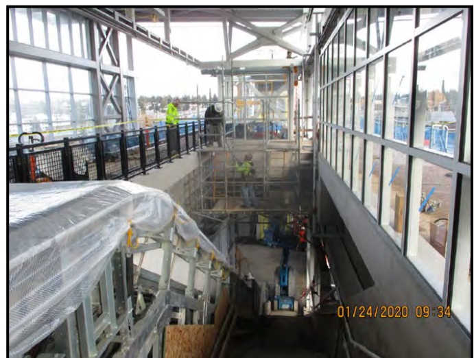
Setting up scaffolding at Stair 1 for closet framing
