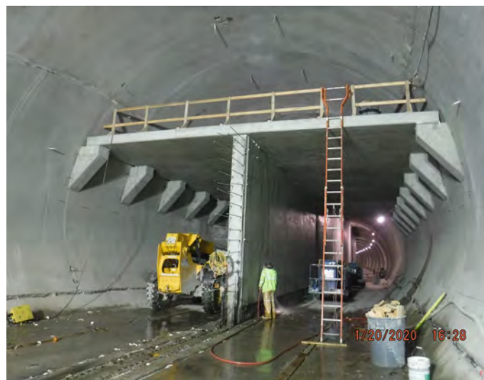
Power wash and cleaning center wall at Expanded Zone.
