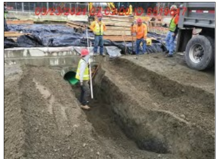
51st Excavation for waterline tie in.
