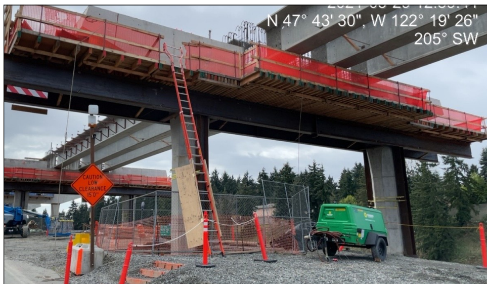
Temporary walkway installation & girder placement
