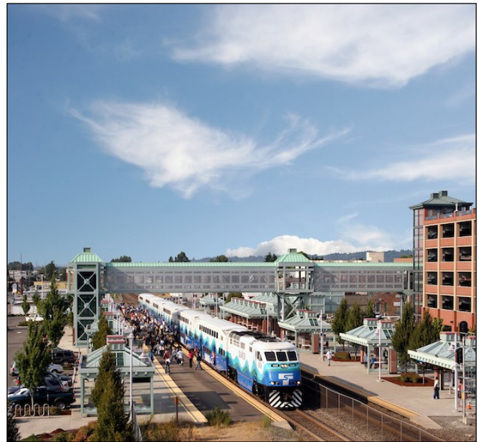
Improving access to Sounder Auburn Station
