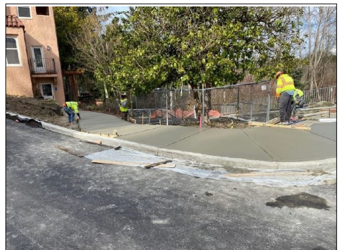
Winters House ADA Sidewalk installation
