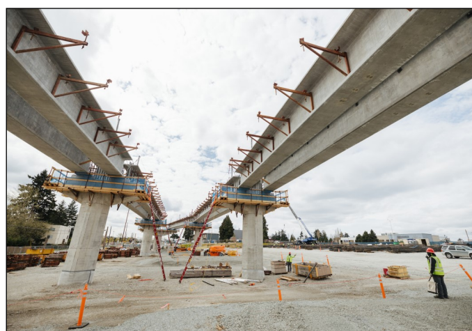
First girders for the project at KDM station area
