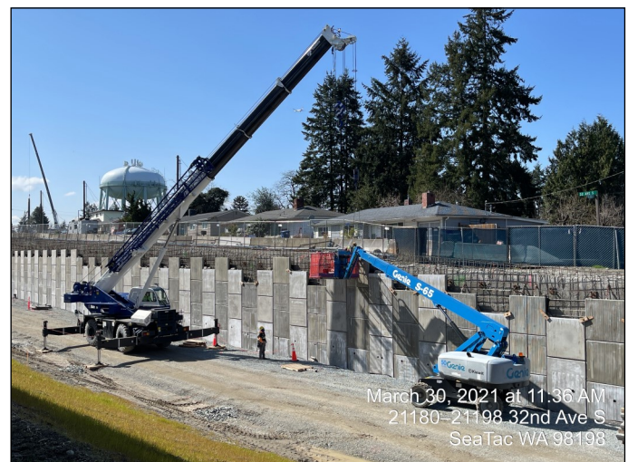
Setting precast wall panels (Wall R1025 in WA1.2)
