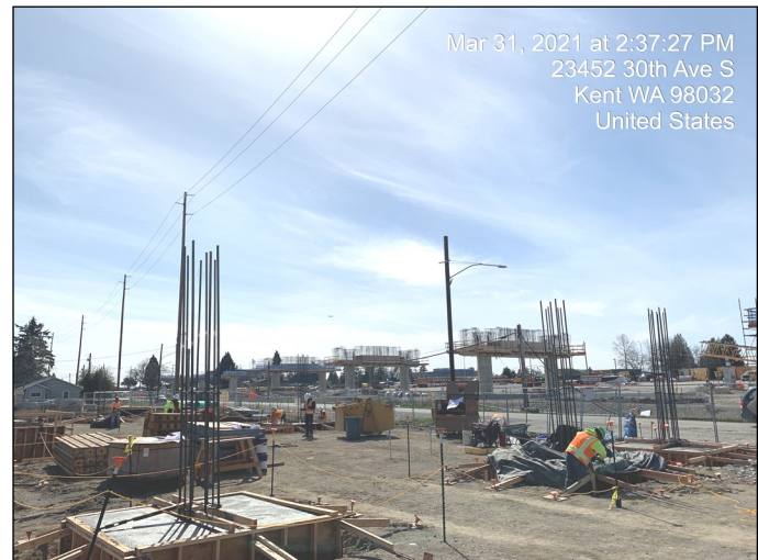
Progress of foundation concrete placement at WAI.3
