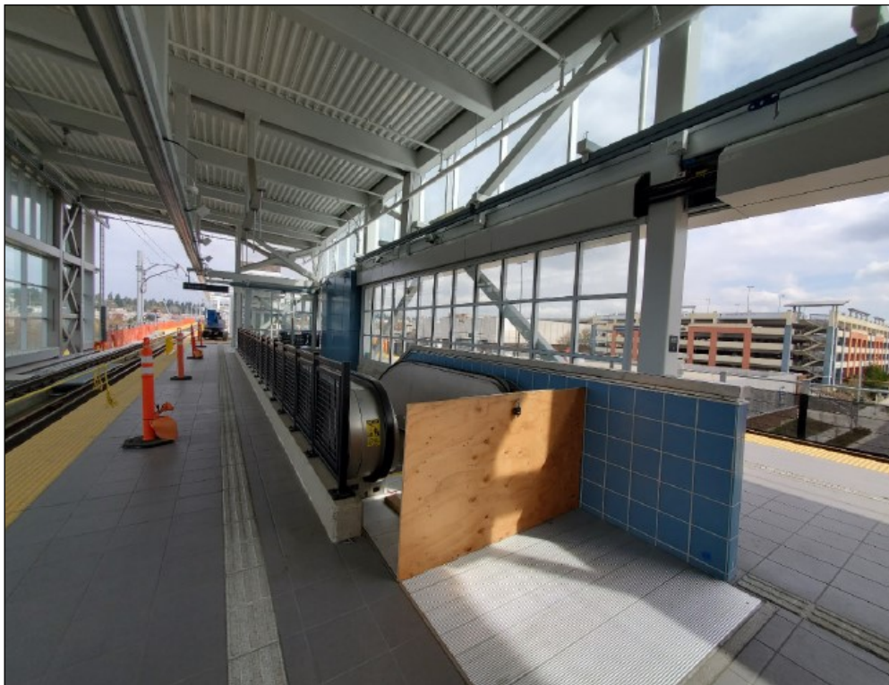
N160—Workers cleaning windows at Northgate Station's South Entry.
