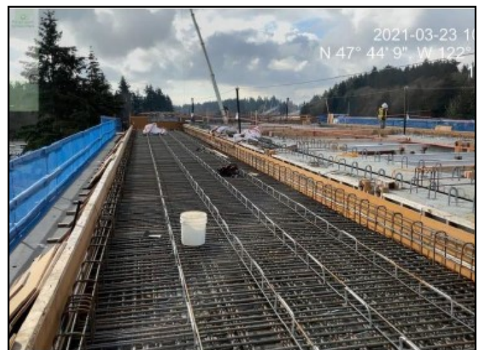
148th station girder span rebar.
