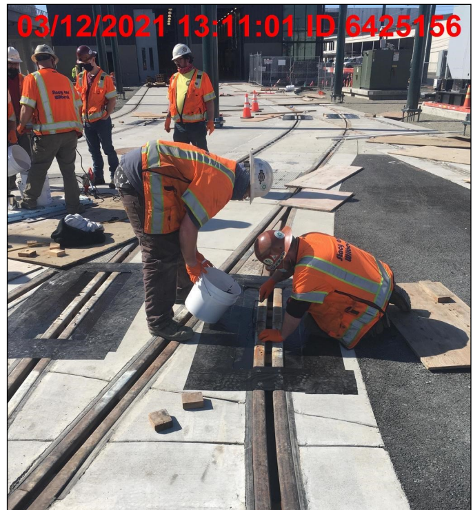
Epoxy gout installation at the OMF
