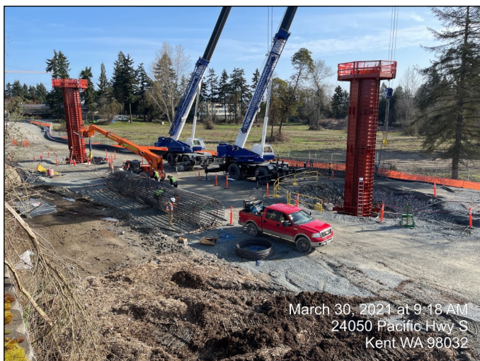
Column reinforcement cage placement (NE at WA2.1)
