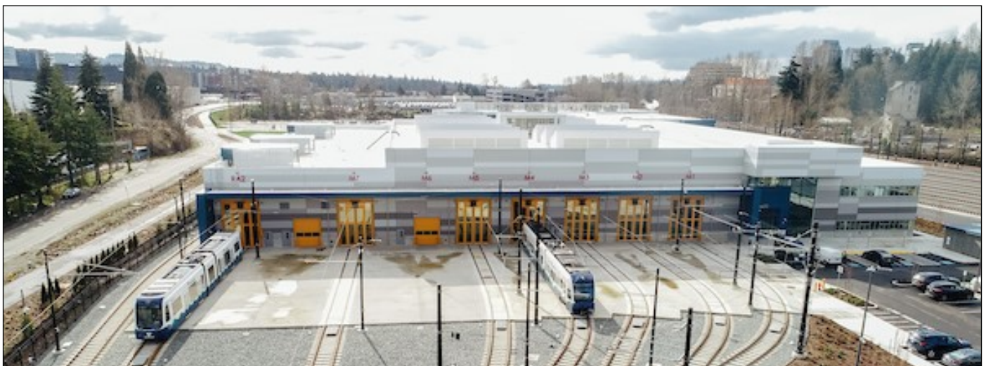
Operations and Maintenance Facility East in Bellevue
