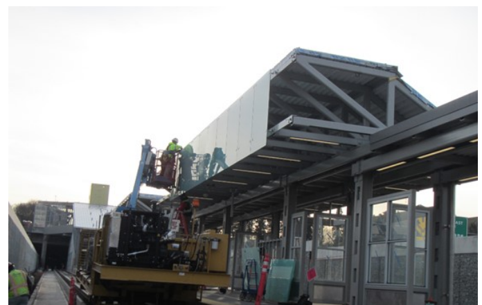
Crews installing glazing — Judkins Park Station, SE platform center canopy
