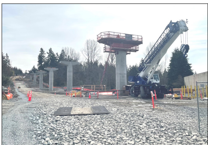
Columns and caps for structure A in SeaTac
