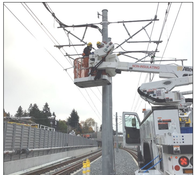
Installing feeder cabling south of Northgate Station.
