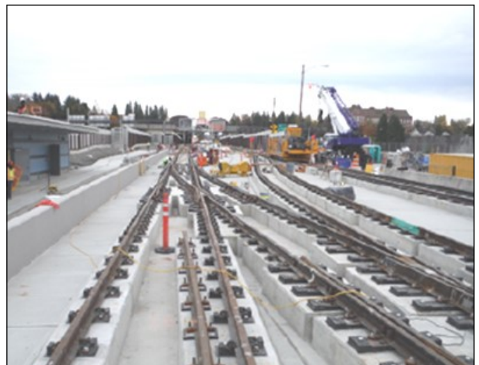
Specialty turnaround track installed at Judkins Park Station
