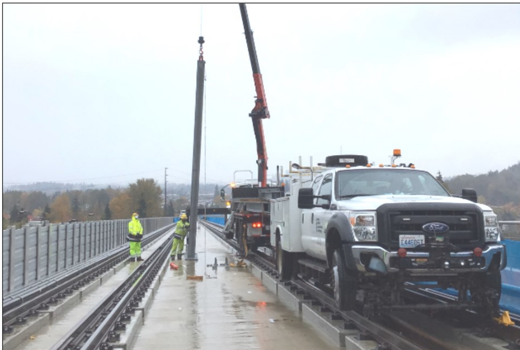
E750 Systems: OCS Pole Installation over E360's elevated guideway near Redmond Technology Station.
