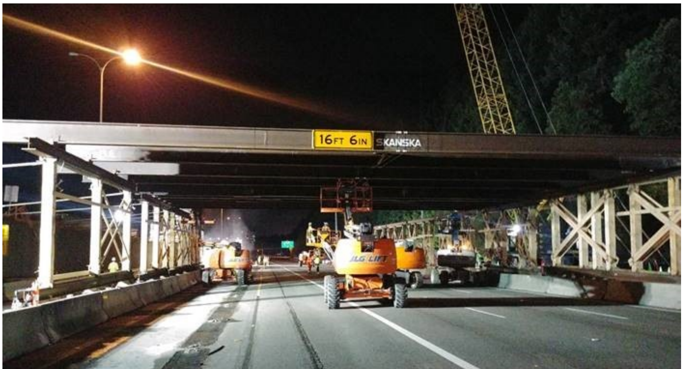
L-300 contractor (Skanska) installing stringer beams that will support our Lynnwood Link bridge over I-5
