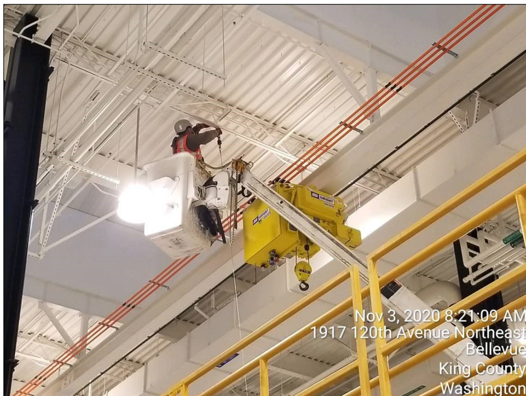
Movement of the Shop OCS Dropper Cable
