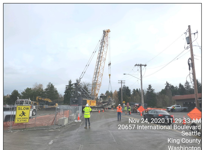
Drill rig mobilization to Structure A
