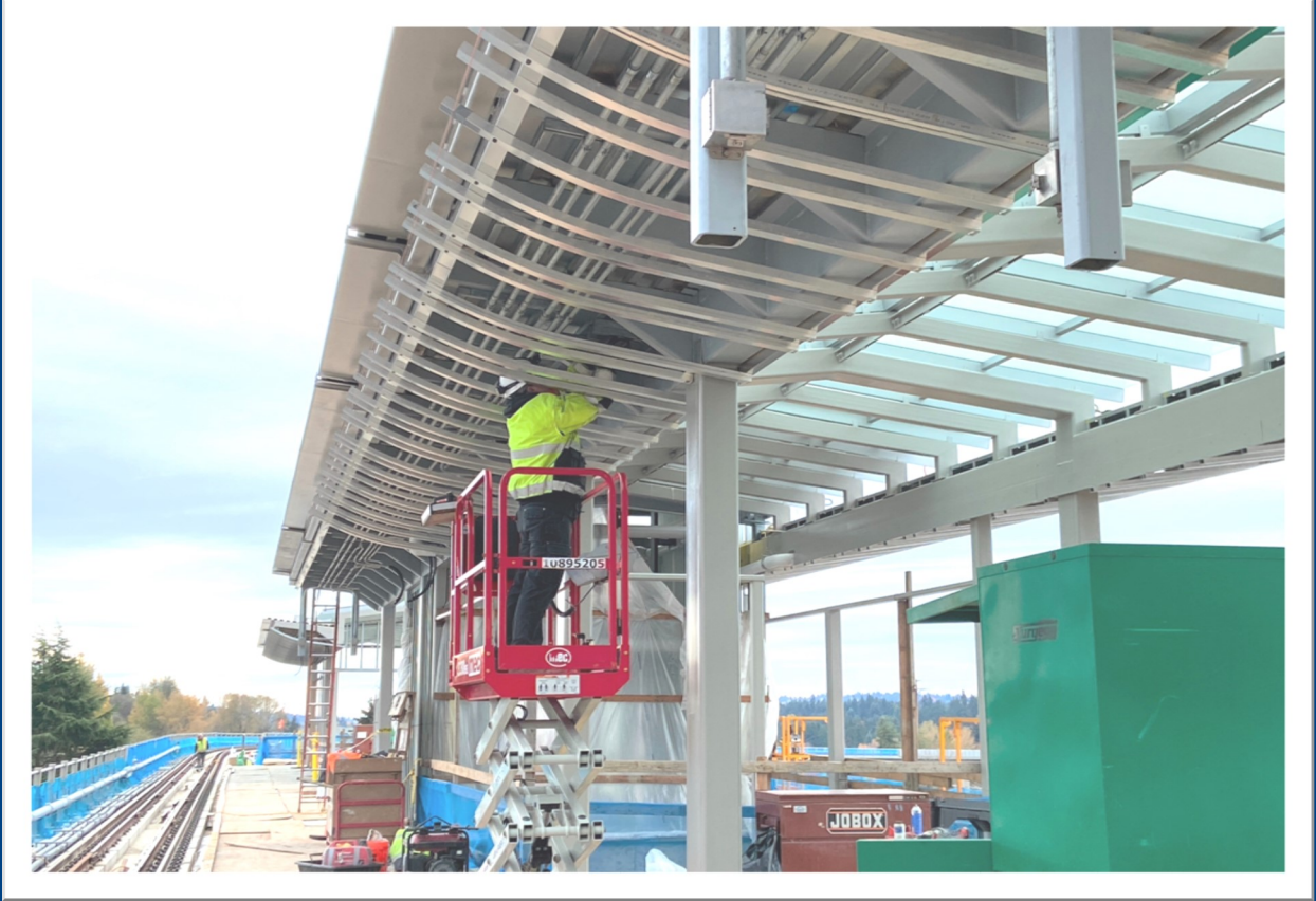
Electrical Rough-in Work on Platform Canopy (East Link Extension)
