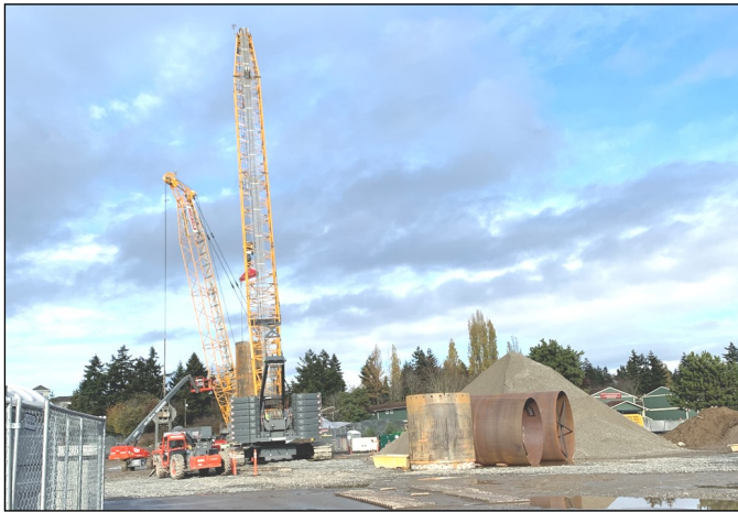
The first drilled shafts in SeaTac
