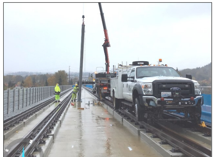
Installation of OCS pole near Overlake Transit Station.
