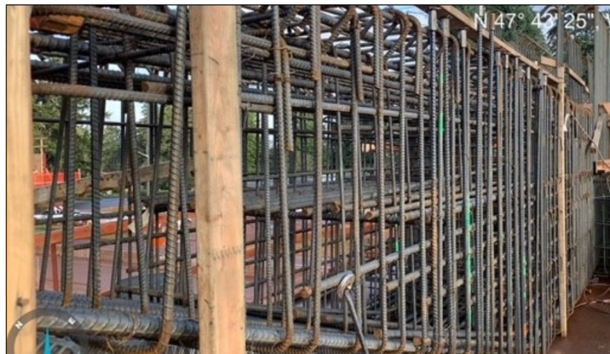
Bent cap reinforcing steel
