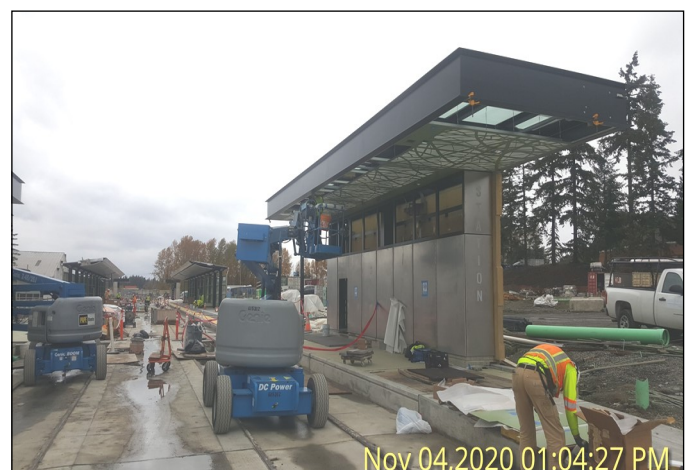
LED lights and conduits installed at northeast entry canopy facing west.
