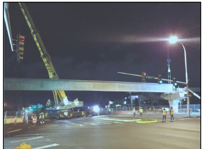
Setting girders between pier H03 and H04 across 220th St.
