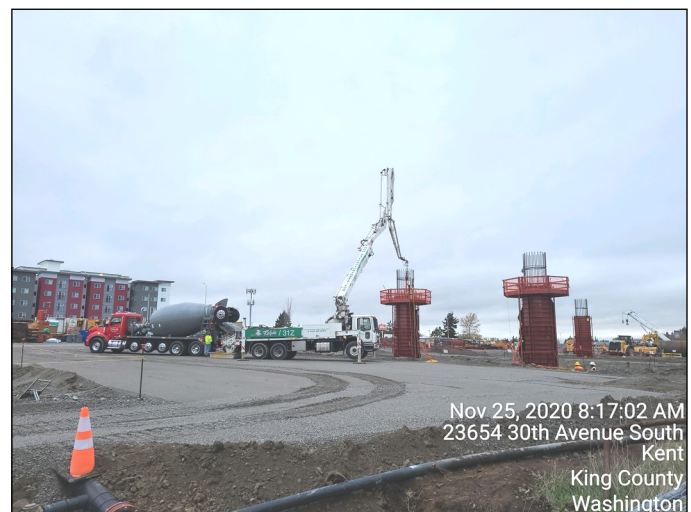
Column B11R (Structure B) concrete placement
