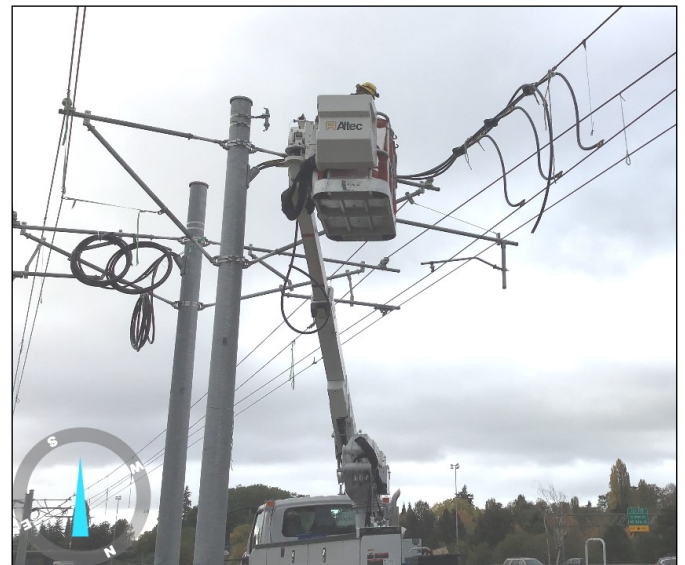
Installation of feeder cable near Northgate Station
