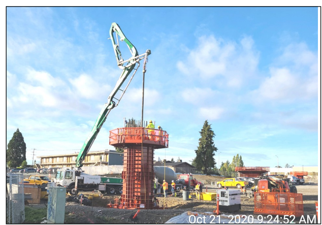
Column concrete placement
