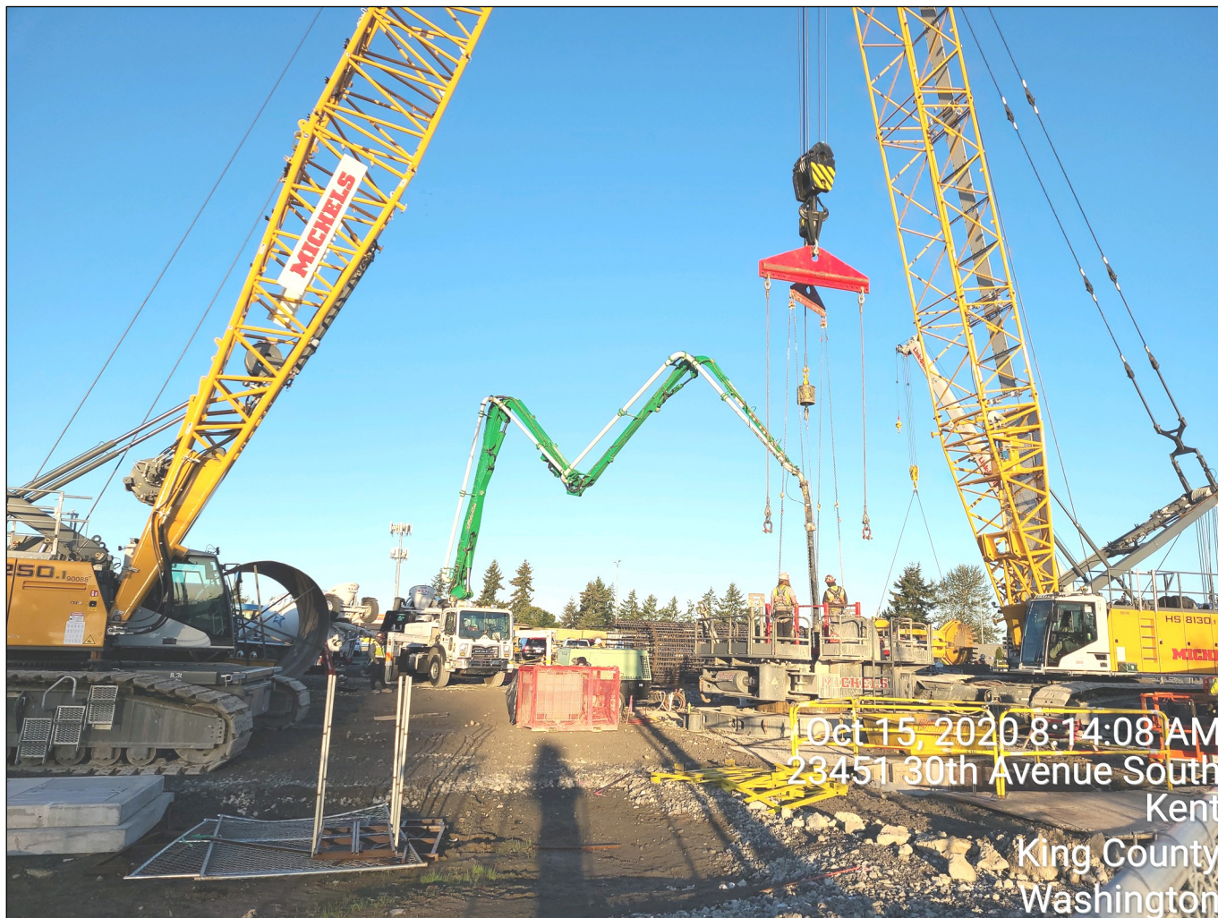
Shaft Concrete Placement (Federal Way Link Extension)
