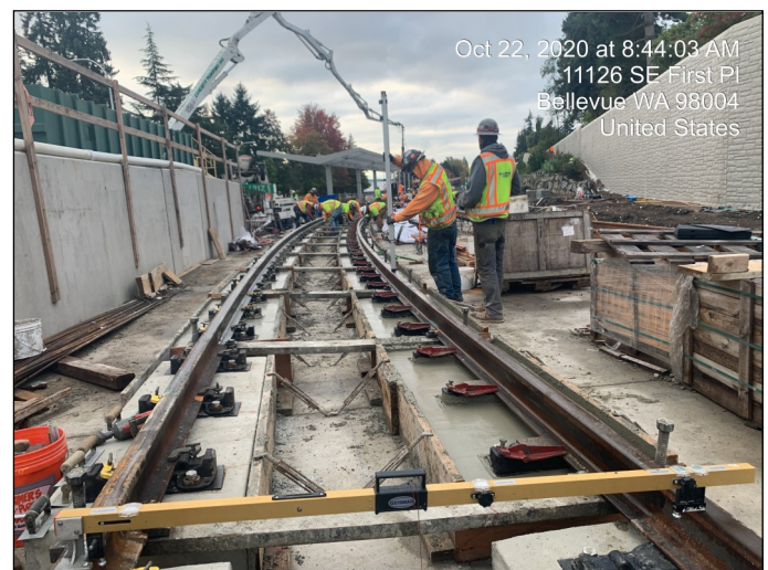
East Main Station: Plinths concrete placement.
