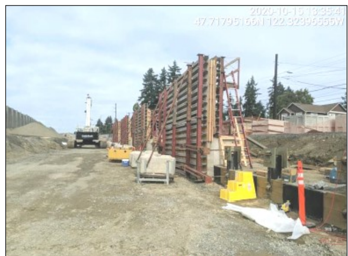
Noise wall construction along I-5
