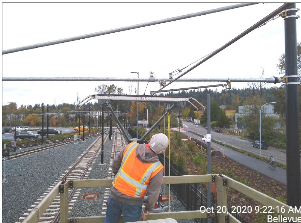
OCS Pantograph security check as part of Systems Integration Testing processes
