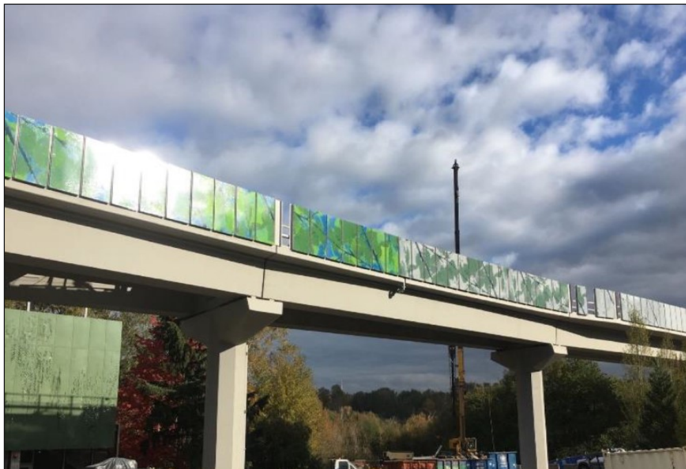
E320 South Bellevue: Functional art — installation of acoustic panels on the elevated guideways.
