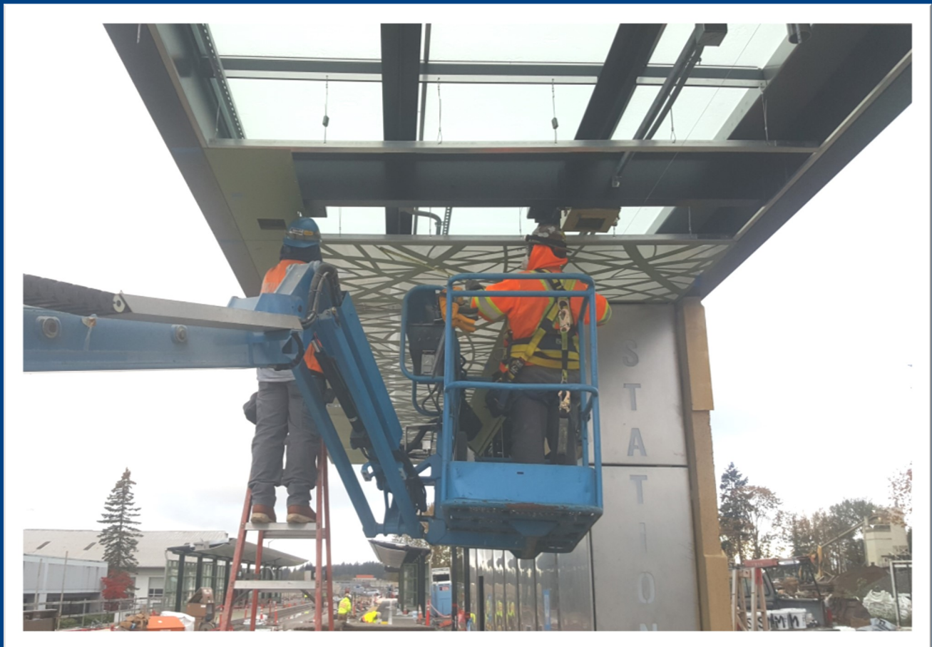
Soffit Panels Installation at the Bel-Red/130th Station (East Link)
