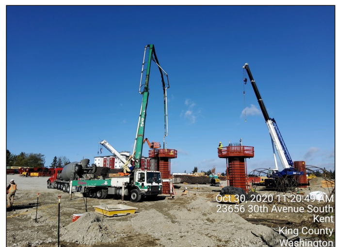
Concrete placement for B14 columns left and right
