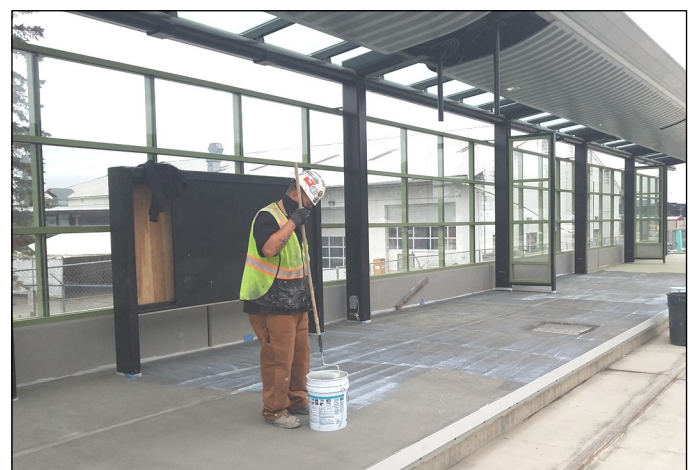
Applying sealer to paver bed at SW-side station platform.
