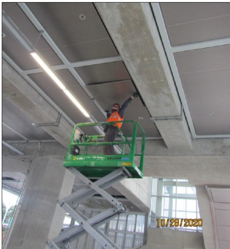
N160—Worker removing ceiling metal panel section at Station for Systems access.
