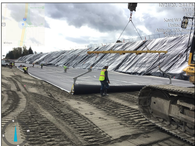
Placement of geomembrane liners at Midway Landfill
