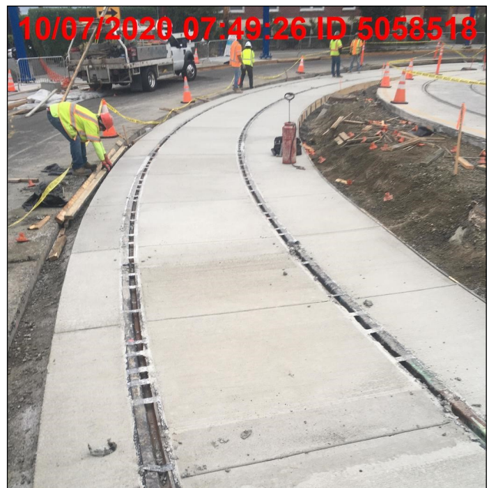
Stripping track slab forms
