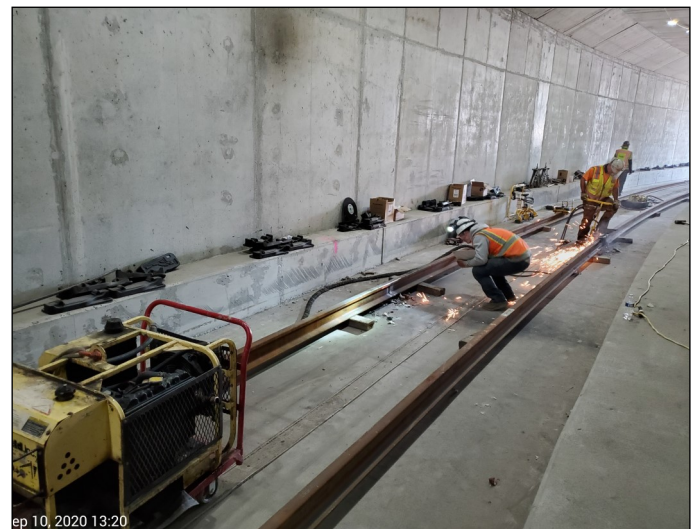
E335 installing tracks at Bellevue Downtown Tunnel.
