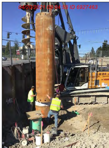
Drilled shaft placing second casing section.
