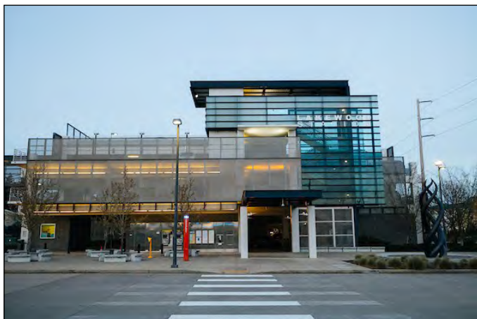
Lakewood Sounder Station Building
