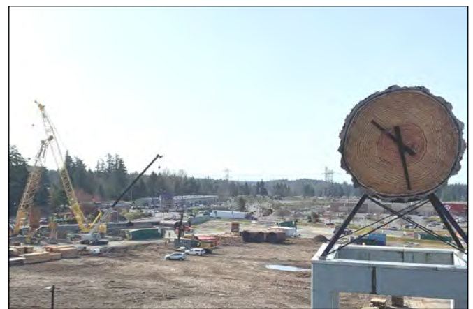
First drilled shafts going in at Federal Way Transit Center
