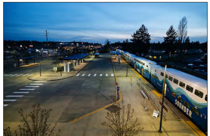
Lakewood Station Passenger Platform Access
