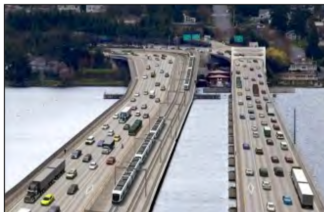
Since June 2017, the project has provided 24/7 HOV access on I-90 between Seattle, Mercer Island and Bellevue.
