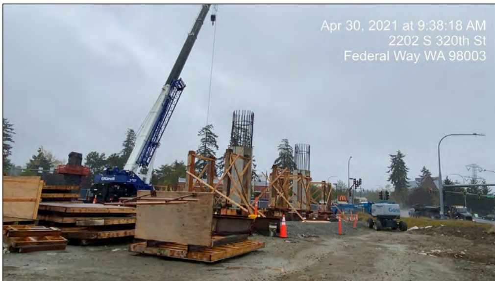
Erection of falsework at Columns G24 (in WA 3.8)
