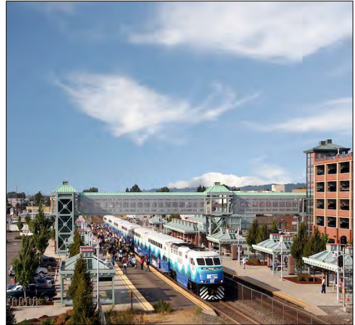
Improving access to Sounder Auburn Station
