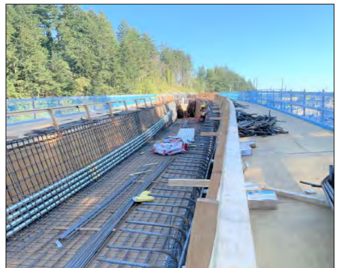
Placing rebar for the I-5 overcrossing.
