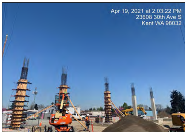
Progress of formwork columns on 30th Ave, Kent
