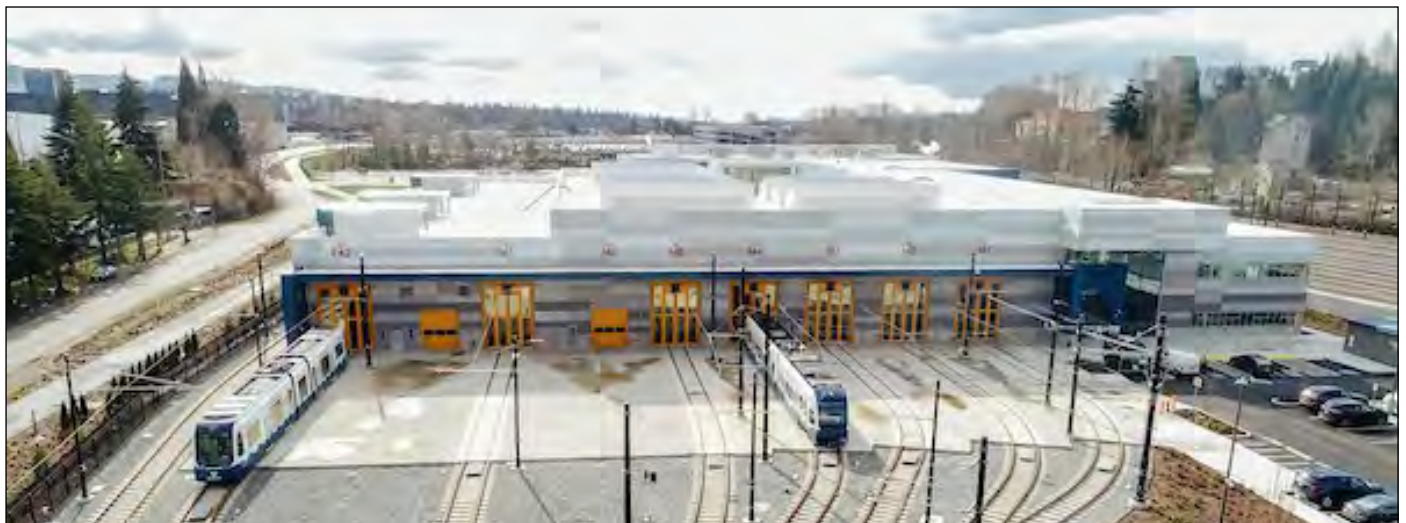
Operations and Maintenance Facility East in Bellevue
