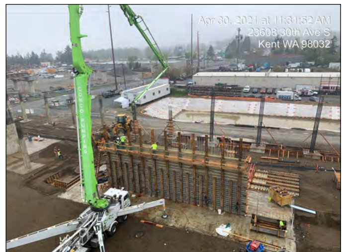
Concrete shear wall placement at KDM
