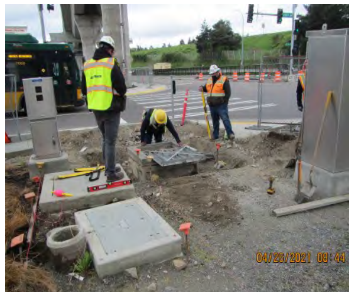
Corner of NE 100 th and 1 st NE Absher Stringing Vault for Lowering
