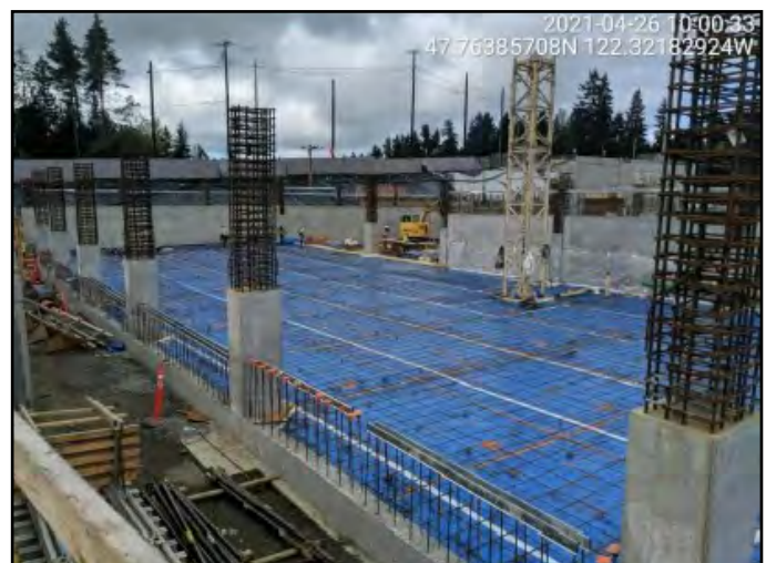
185th garage slab on grade rebar installation
