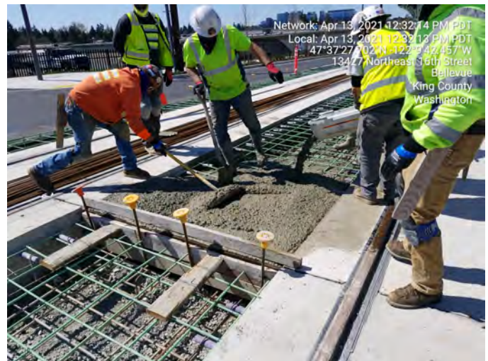
Placing concrete in the center track slab facing west.
