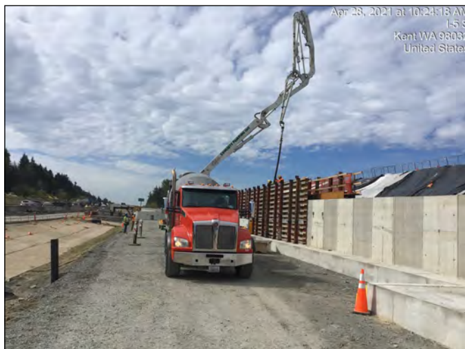
Midway Landfill concrete placement for cast-in-place wall
