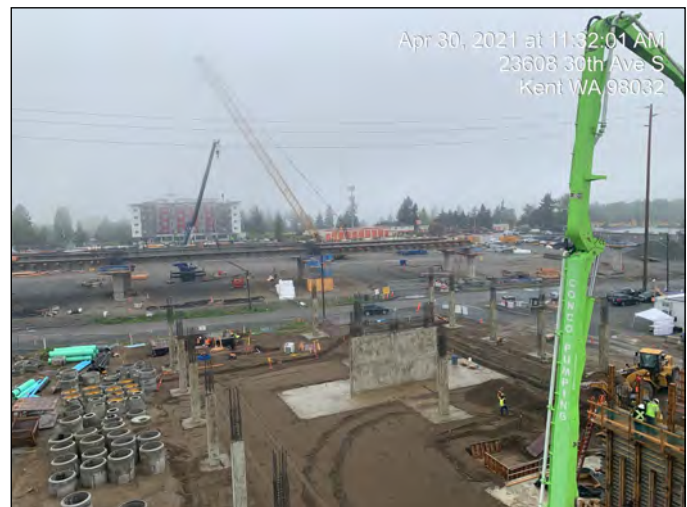
Progress at the KDM Station site.
