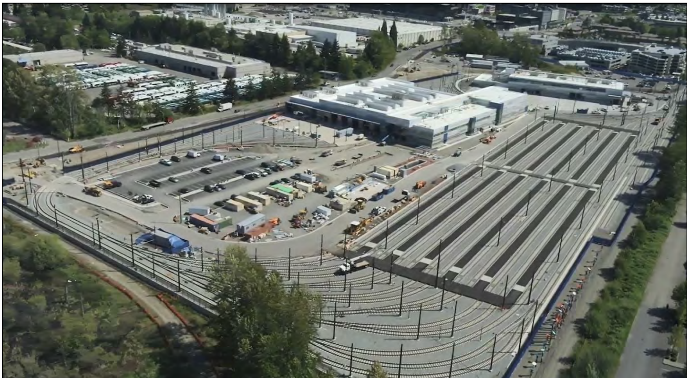
OMF East - OMF Building (front) and MOW Building (back) and STart Nails (lower right) along the Maintenance Yard
