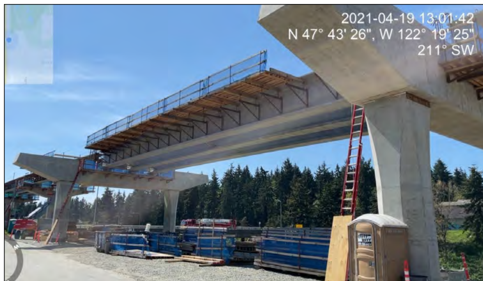
girder span placement
